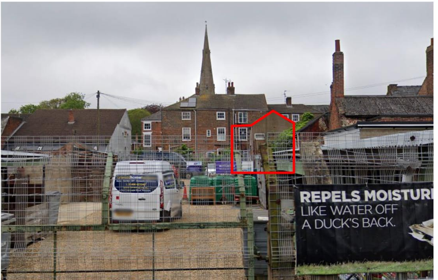
View of the rear of the property from Chapel Street
