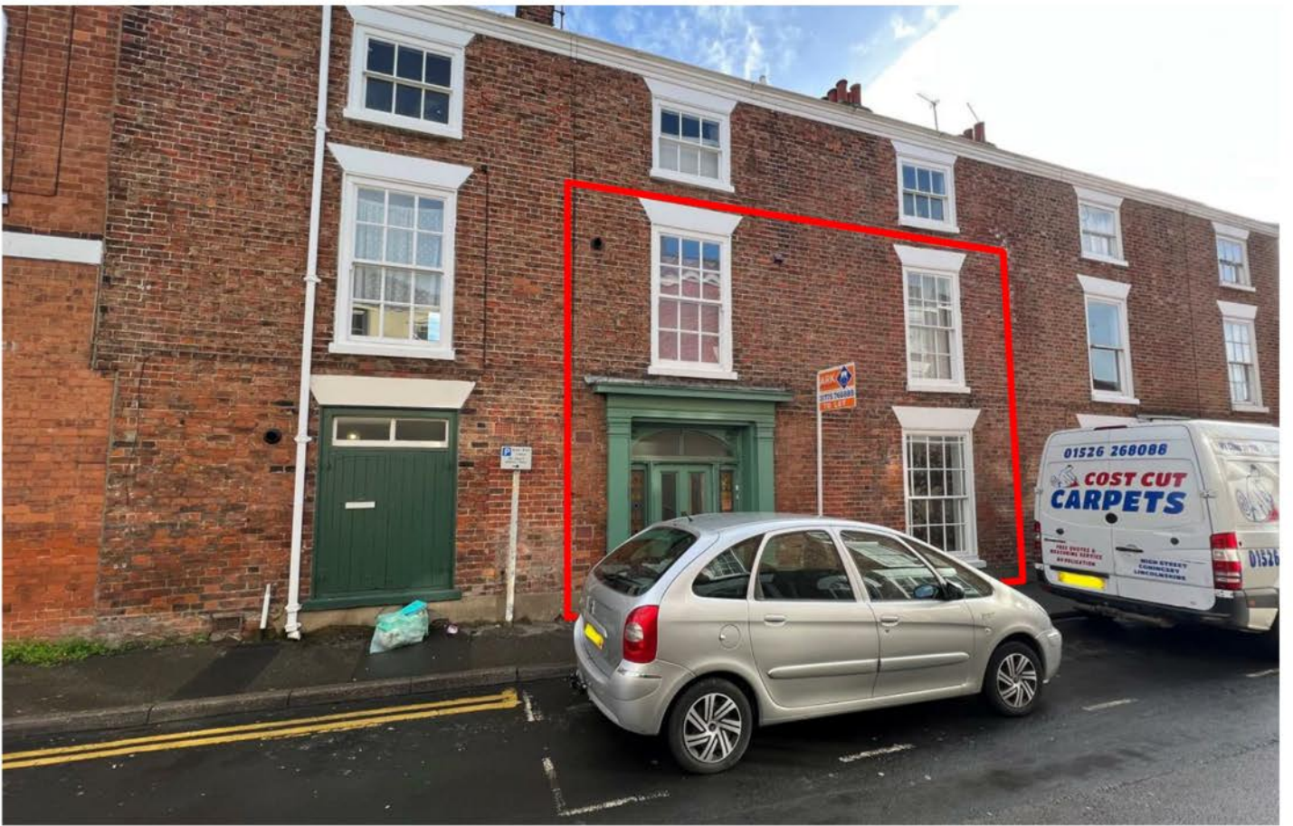
View of the front of the property from Albert Street
