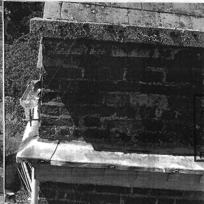
South west corner parapet.
