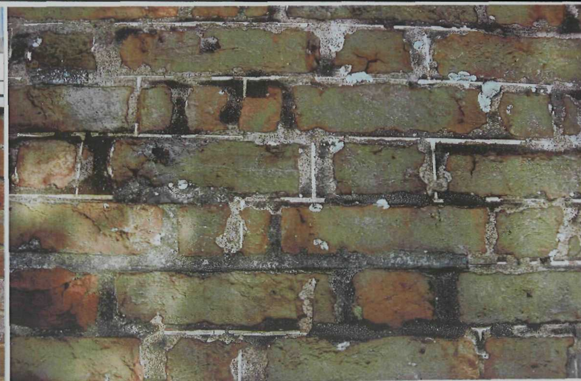
E. elevation "tuck pointing".
