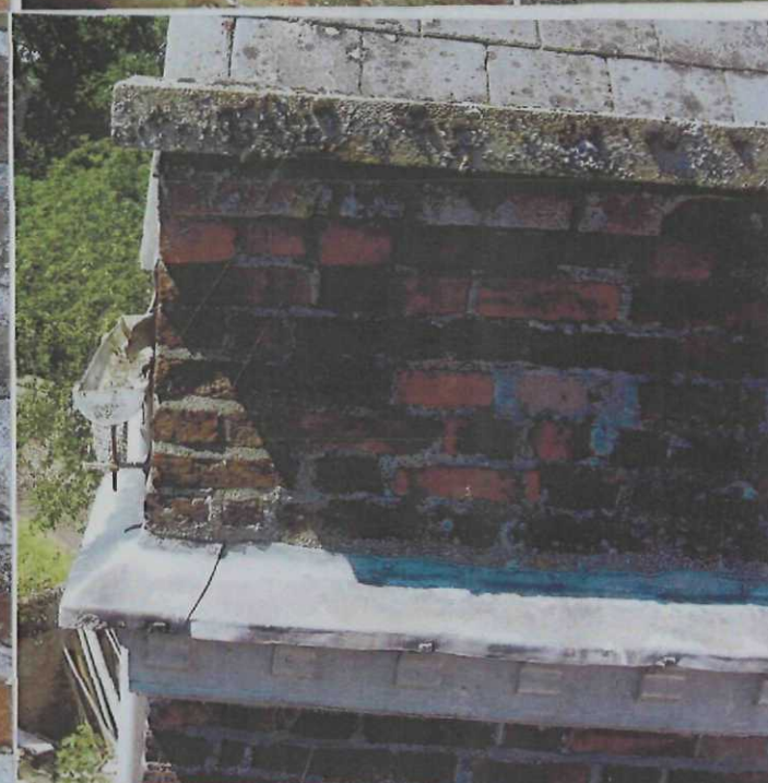
South west corner parapet.
