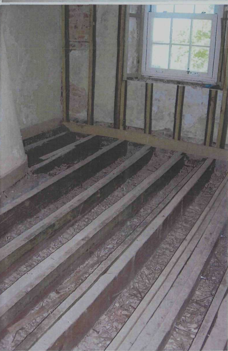
first floor-east Room #F
