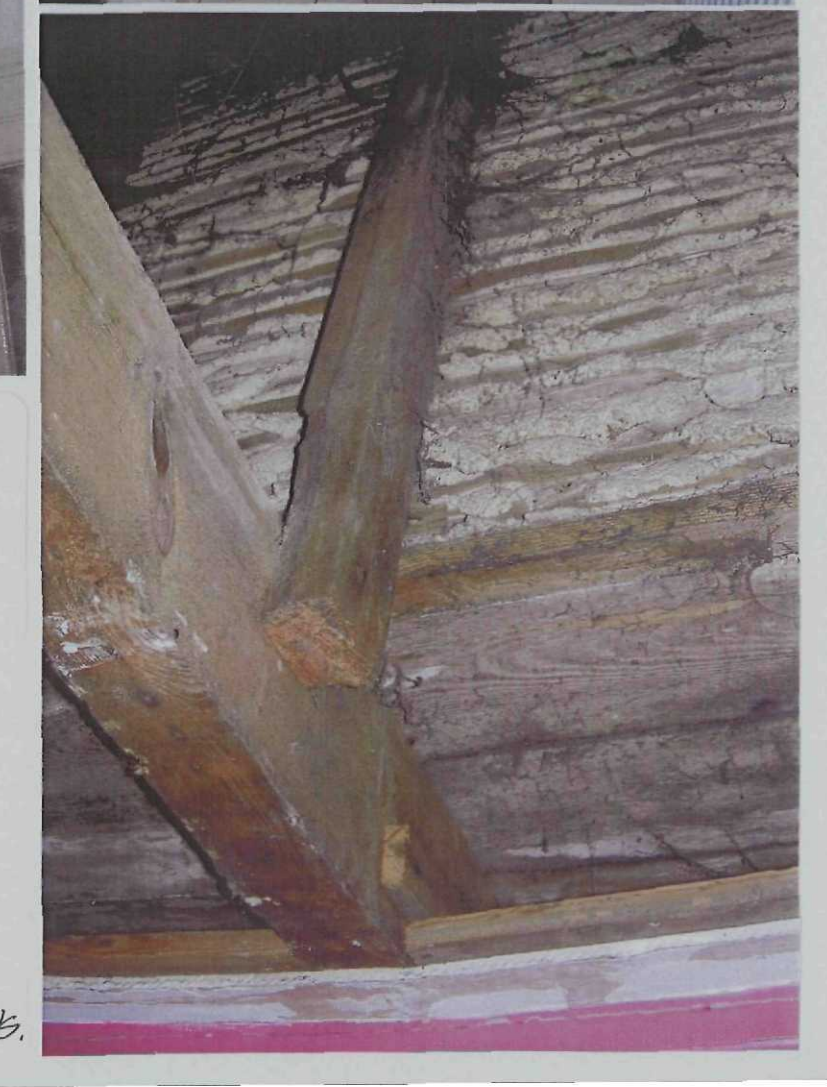
Staircase Landing FF-
