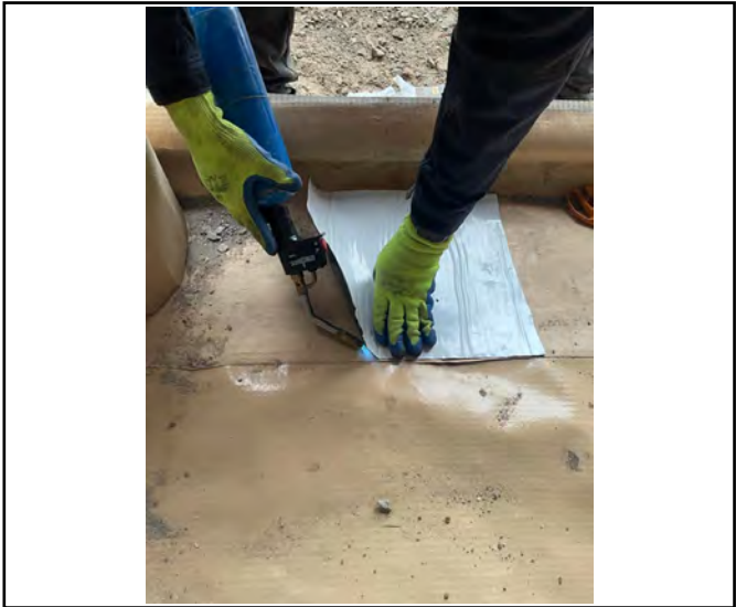
Gas blow torch used to aid in adherence of PAG SAGR.
