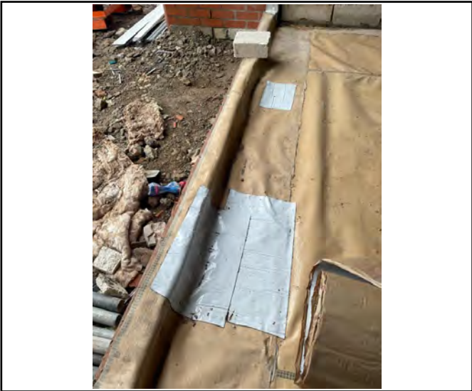
Additional patch repairs carried out using PAG SAGR.
