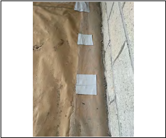
Additional patch repairs carried out.
