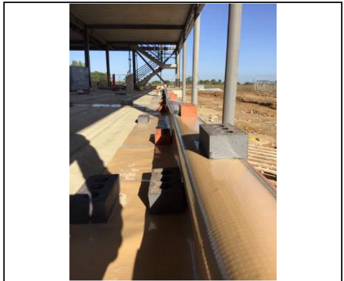
Membrane installed across proposed cavity.
