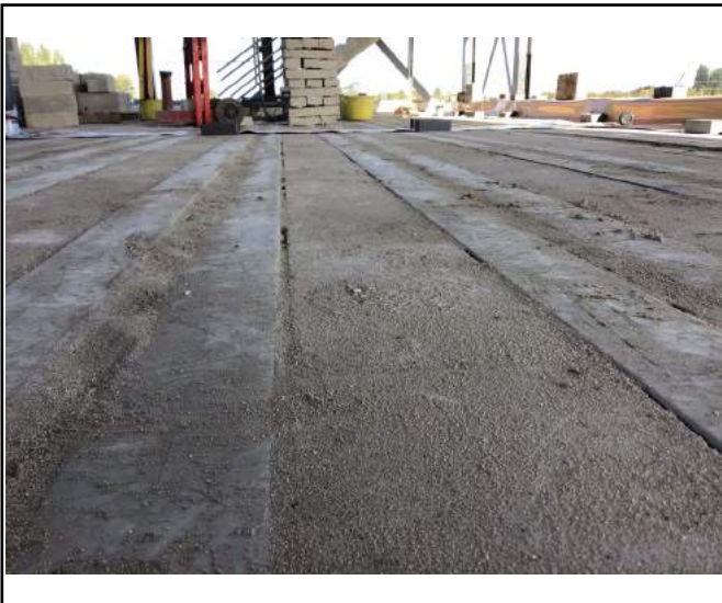
Smooth block and beam floor
