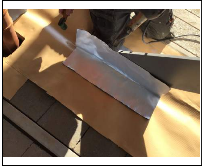
Installer applied PAG SAGR to a steel
