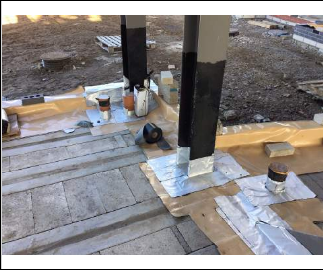
Overview of sealed pipes and steel
