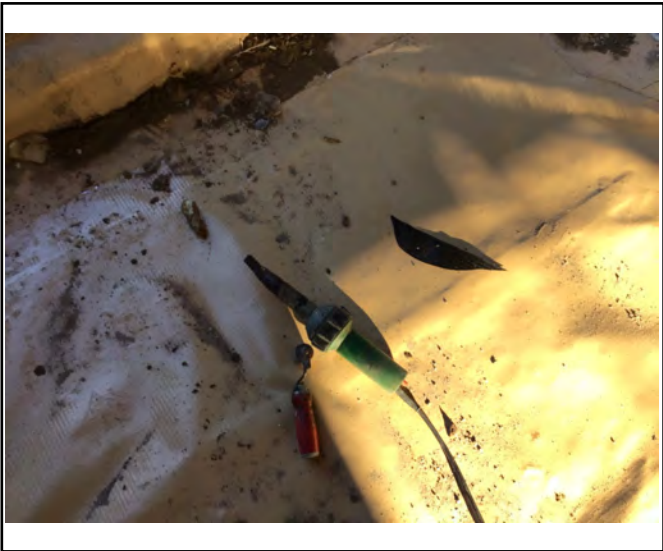
Leister and roller used during install
