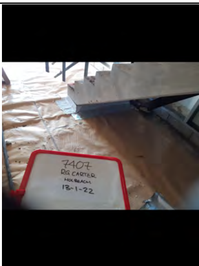
Sealed stair well
