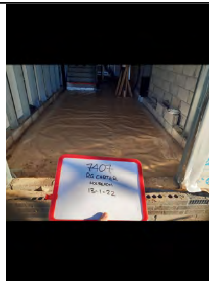
Sealed stair well
