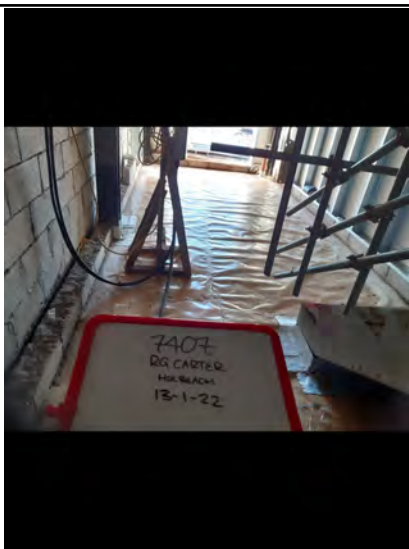
Sealed stair well
