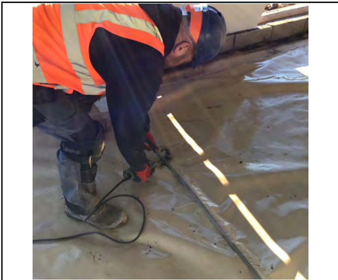
Remediation of lap joint
