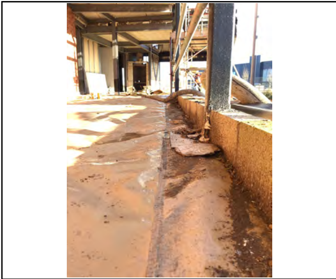
Infill terminated to perimeter membrane
