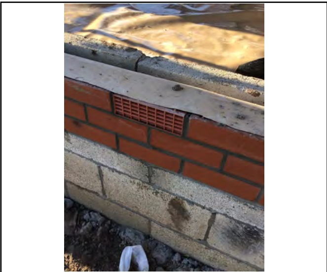
Air brick in perimeter
