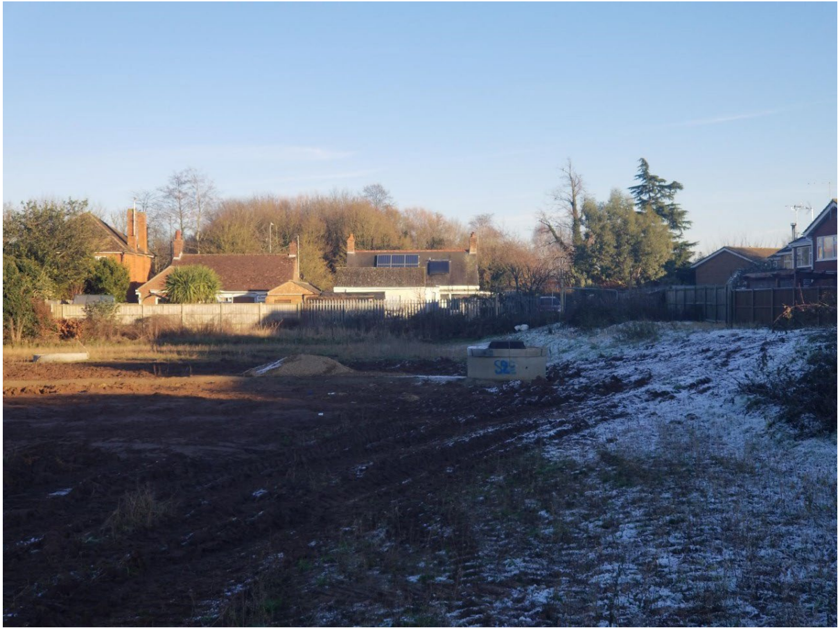
PLOT 62 (ELM DRIVE – MANHOLE)
