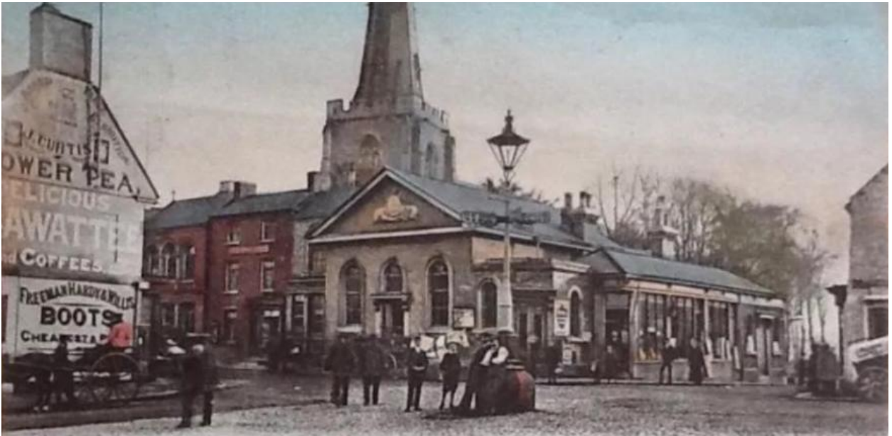
Figure 8 Presumed late 19 th century photograph with the study area former building to the far right of the image. 9
