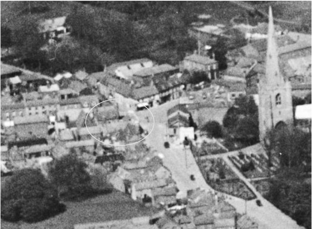
Figure 16 Extract from a 1930 aerial photograph looking north with the site circled. 19 No first floor structure was suggested in 1930.
