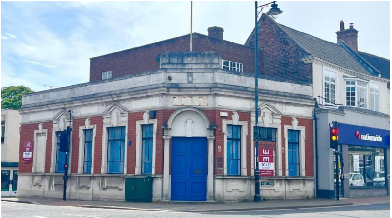
Figure 24 Looking southwest to the northeast corner of 1 West End in c.2024. 28
