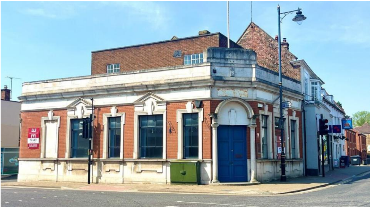
Figure 23 Looking southwest to the northeast corner of 1 West End in c.2024. 27
