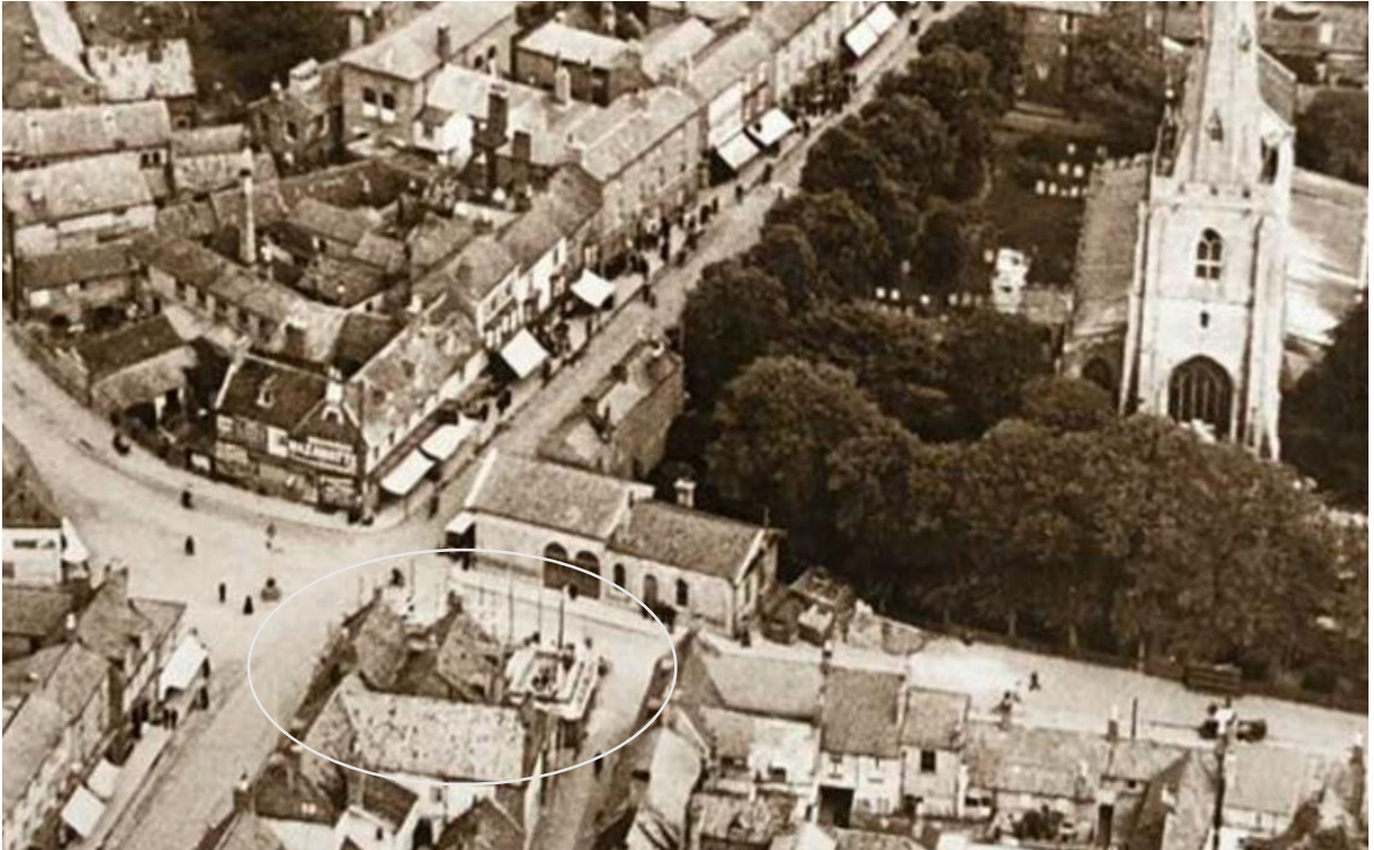
Figure 12 c.1922 aerial photograph showing the study area left of centre in the lower part of the image. 15 It would appear to show scaffolding poles erected around the east and north sides of the building in this image and likely the time of construction of the original building.
