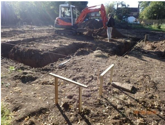
Plate 49: Excavation of the foundations, from the north
