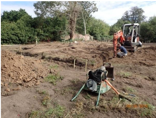
Plate 54: Excavation of the foundations, from the west
