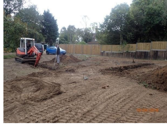
Plate 62: Excavation of the foundations, from the north-west
