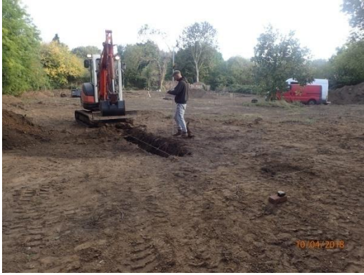
Plate 59: Excavation of the foundations, from the south
