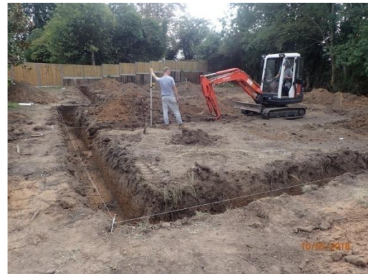
Plate 99: Excavation of the foundations, from the north
