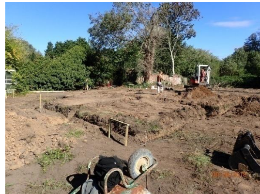
Plate 57: Excavation of the foundations, from the south-west
