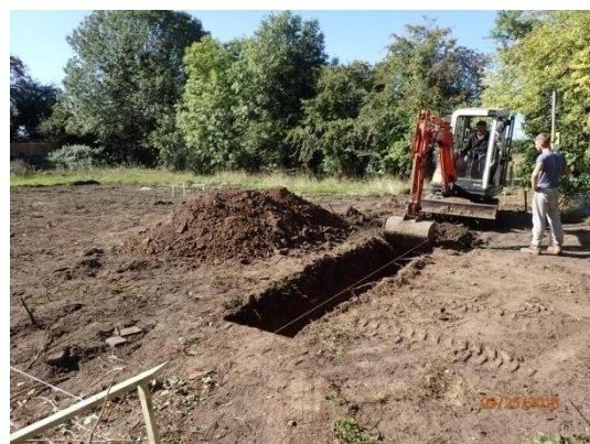
Plate 34: Excavation of the foundations, from the east
