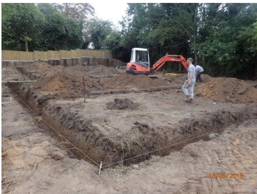
Plate 103: Excavation of the foundations, from the north
