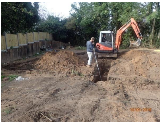
Plate 85: Excavation of the foundations, from the south
