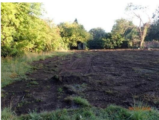
Plate 31: Pre-groundworks, from the south
