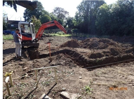
Plate 44: Excavation of the foundations, from the north
