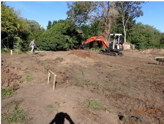
Plate 42: Excavation of the foundations, from the south
