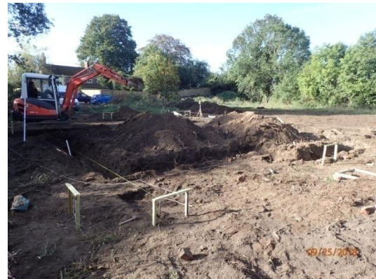
Plate 21: Excavation of the foundations, from the north-east
