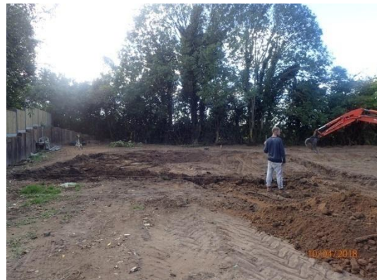
Plate 76: Excavation of the foundations, from the east
