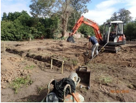
Plate 53: Excavation of the foundations, from the west
