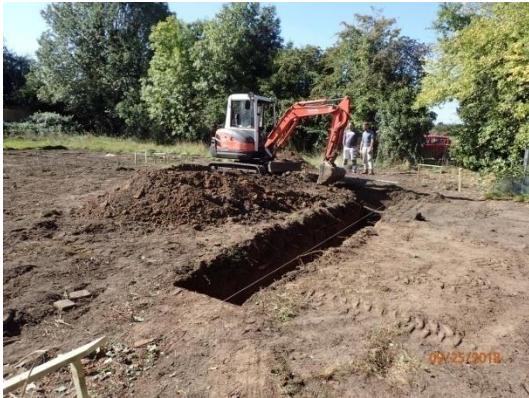
Plate 36: Excavation of the foundations, from the east
