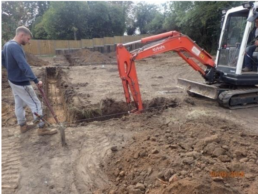
Plate 90: Excavation of the foundations, from the north
