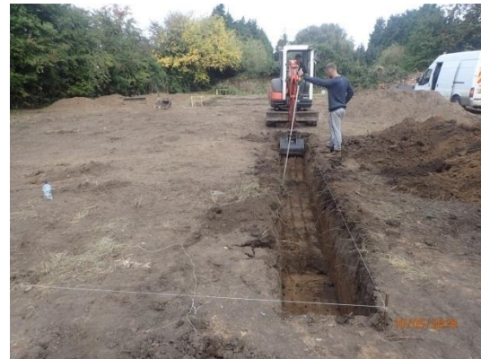
Plate 87: Excavation of the foundations, from the south
