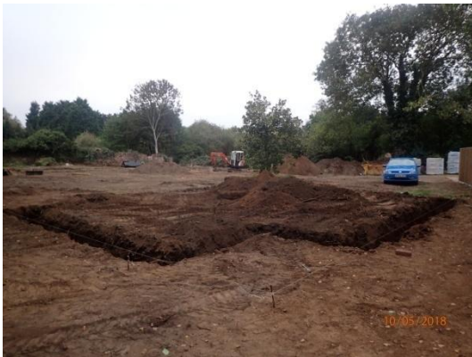
Plate 78: Excavation of the foundations, from the south-west
