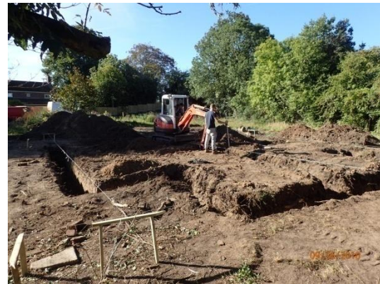
Plate 52: Excavation of the foundations, from the north
