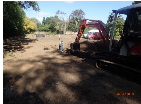
Plate 69: Excavation of the foundations, from the south
