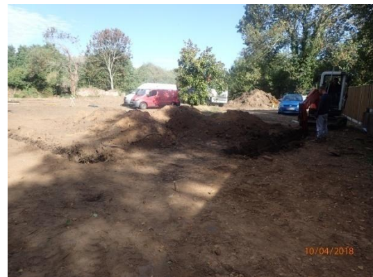
Plate 70: Excavation of the foundations, from the west
