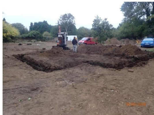
Plate 82: Excavation of the foundations, from the south-west
