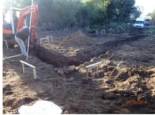
Plate 14: Excavation of the foundations, from the north-west
