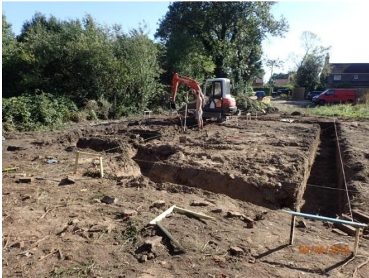
Plate 24: Excavation of the foundations, from the north
