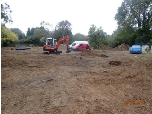
Plate 65: Backfilled trenches, from the south-west
