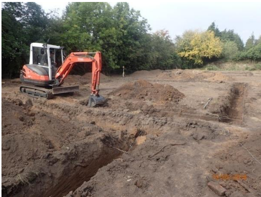
Plate 96: Excavation of the foundations, from the west
