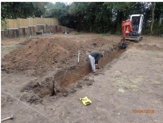
Plate 67: Excavation of the foundations, from the north-east
