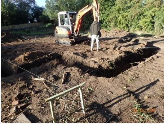
Plate 47: Excavation of the foundations, from the north-east
