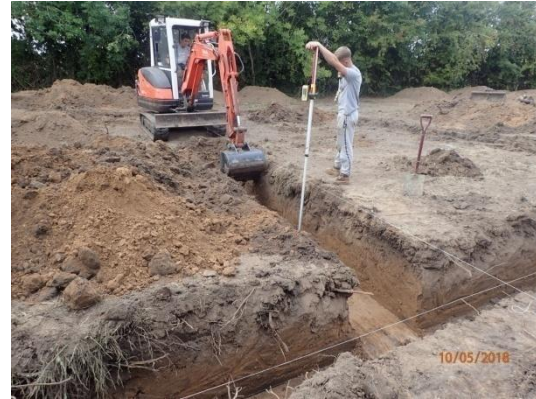
Plate 98: Excavation of the foundations, from the east
