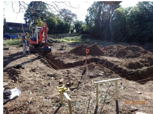
Plate 45: Excavation of the foundations, from the north
