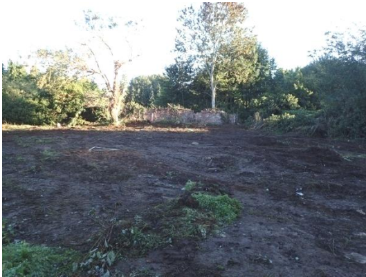
Plate 1: Pre-groundworks, from the south
