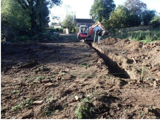
Plate 7: Excavation of the foundations, from the north
