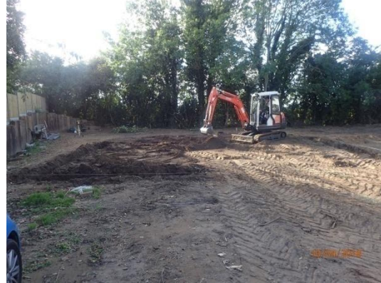
Plate 74: Excavation of the foundations, from the east
