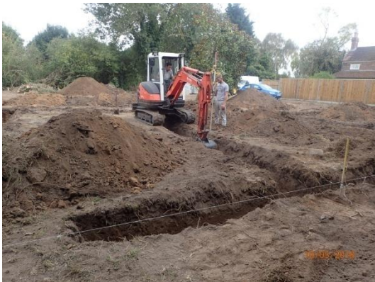
Plate 102: Excavation of the foundations, from the west
