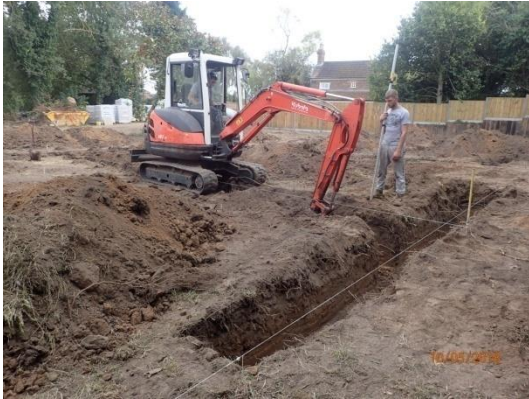
Plate 101: Excavation of the foundations, from the north-west
