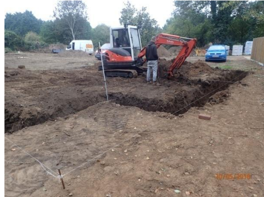
Plate 80: Excavation of the foundations, from the south-west
