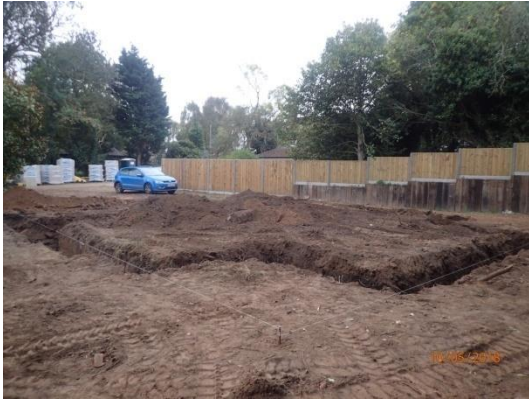
Plate 77: Excavation of the foundations, from the west
