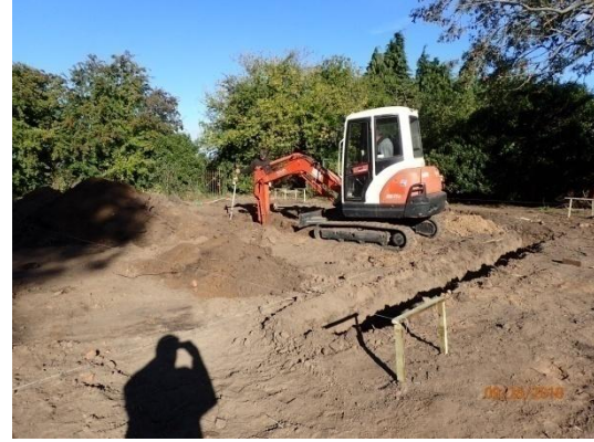
Plate 50: Excavation of the foundations, from the north-east
