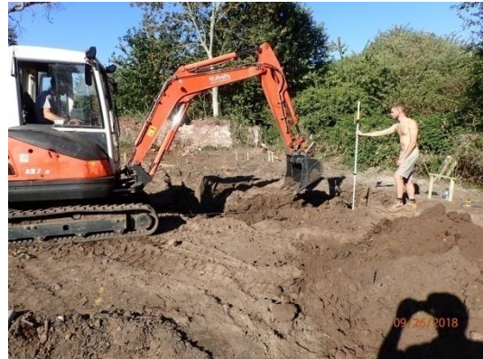
Plate 27: Excavation of the foundations, from the south-east
