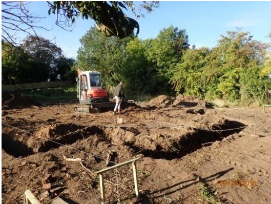
Plate 48: Excavation of the foundations, from the north-east
