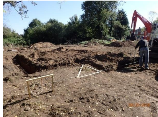
Plate 39: Excavation of the foundations, from the west
