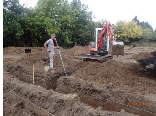
Plate 104: Excavation of the foundations, from the south
