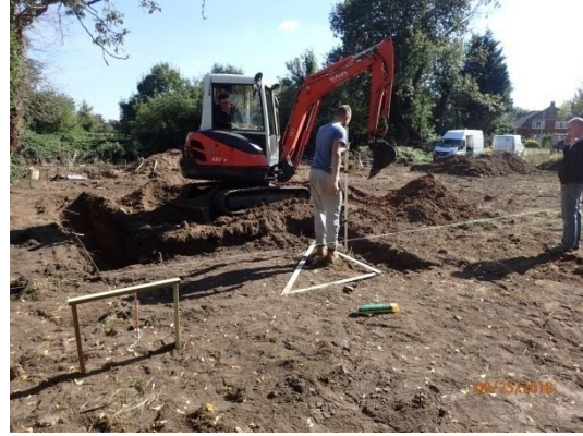
Plate 38: Excavation of the foundations, from the west
