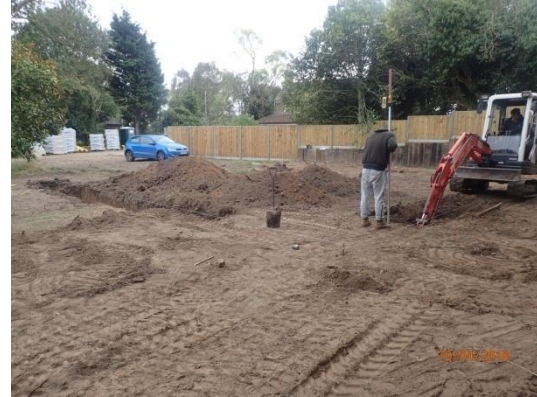
Plate 68: Excavation of the foundations, from the east
