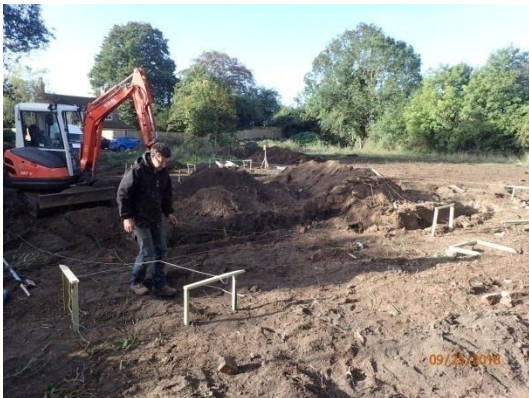
Plate 18: Excavation of the foundations, from the north-east
