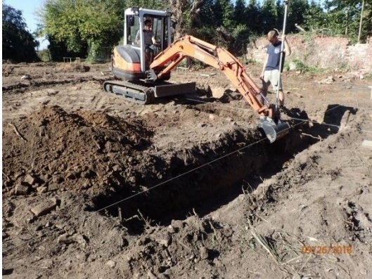
Plate 23: Excavation of the foundations, from the south-east
