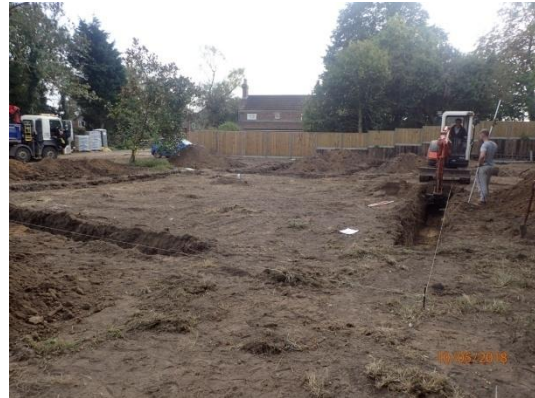
Plate 93: Excavation of the foundations, from the north-west
