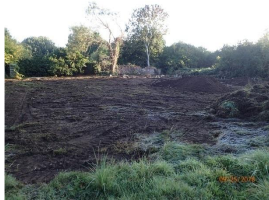
Plate 32: Pre-groundworks, from the south
