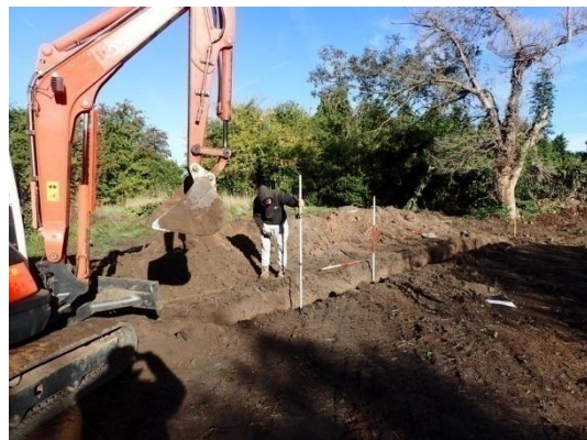
Plate 6: Excavation of the foundations, from the south
