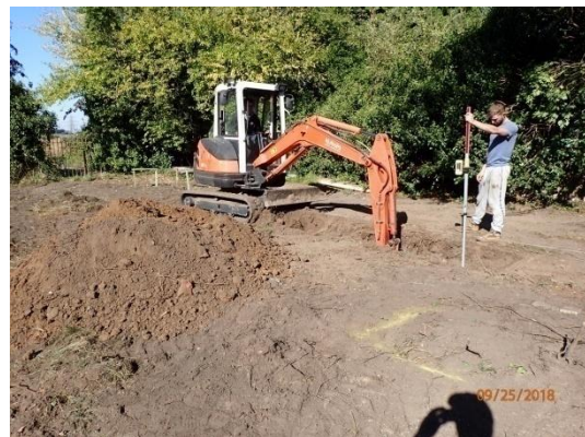
Plate 33: Excavation of the foundations, from the south-east
