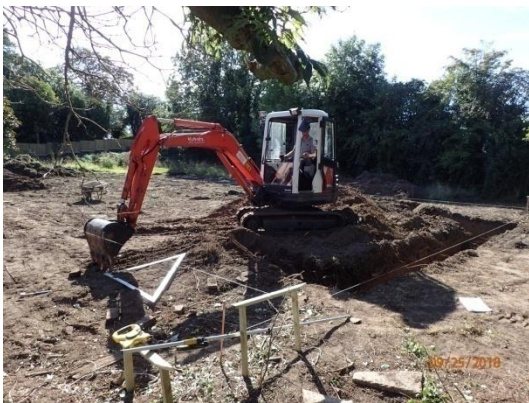
Plate 43: Excavation of the foundations, from the north
