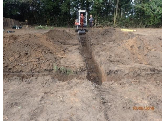
Plate 86: Excavation of the foundations, from the south
