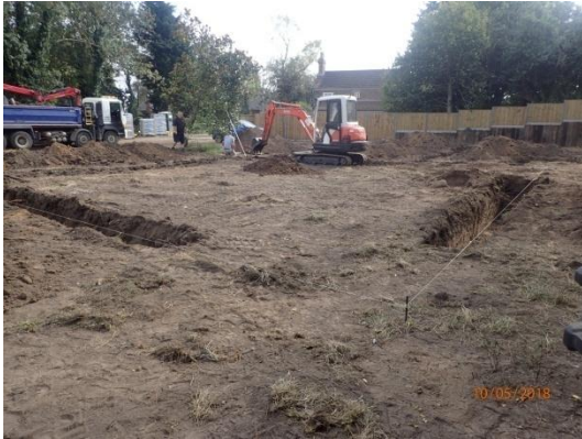
Plate 95: Excavation of the foundations, from the north-west
