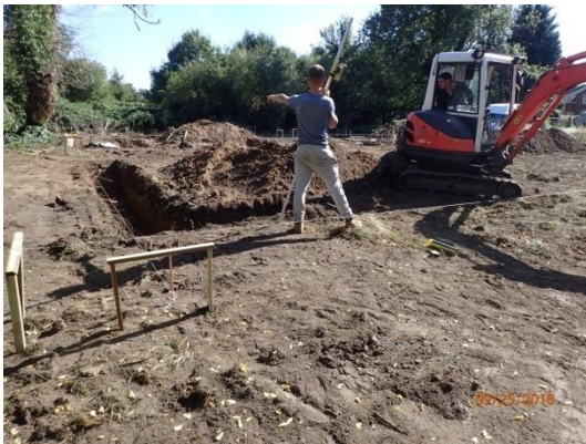
Plate 37: Excavation of the foundations, from the west
