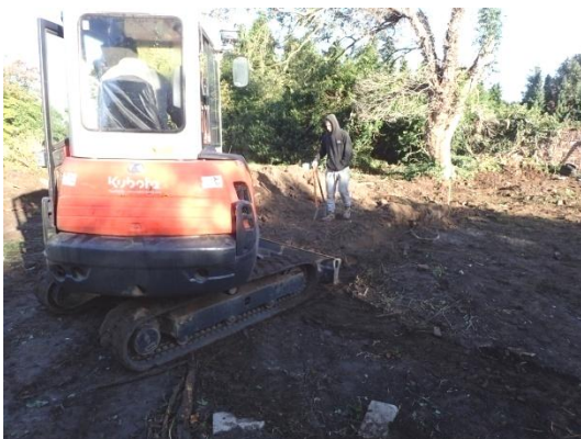
Plate 3: Excavation of the foundations, from the south
