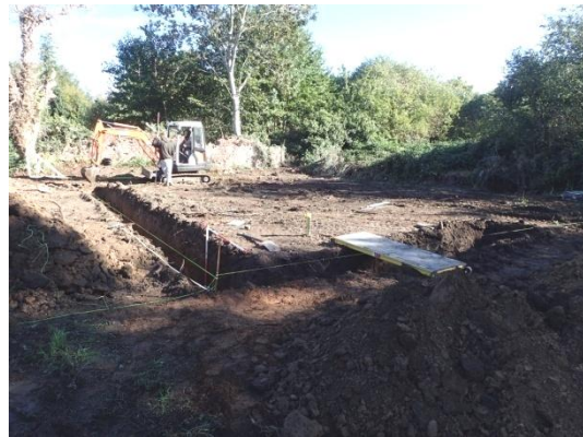
Plate 10: Excavation of the foundations, from the north
