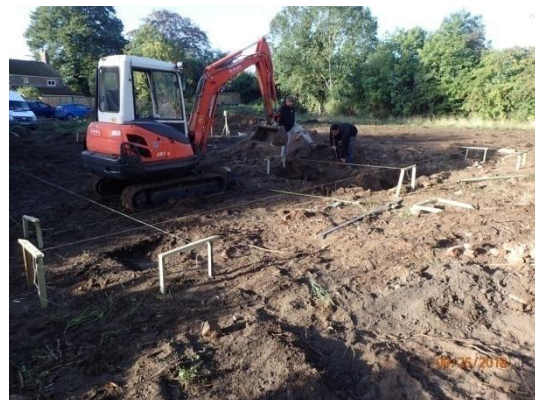
Plate 16: Excavation of the foundations, from the north-east
