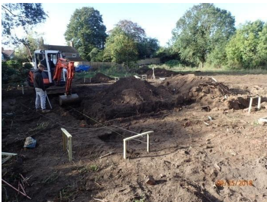
Plate 19: Excavation of the foundations, from the north-east
