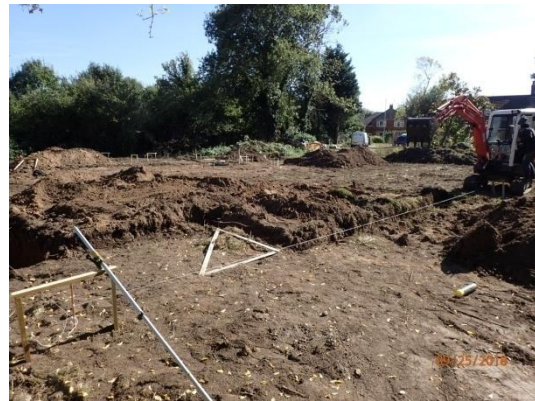
Plate 40: Excavation of the foundations, from the west
