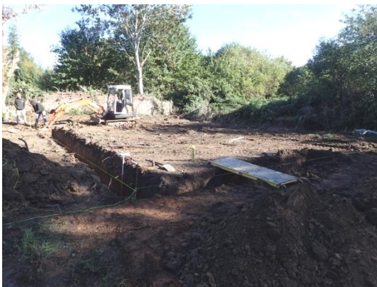
Plate 13: Excavation of the foundations, from the south
