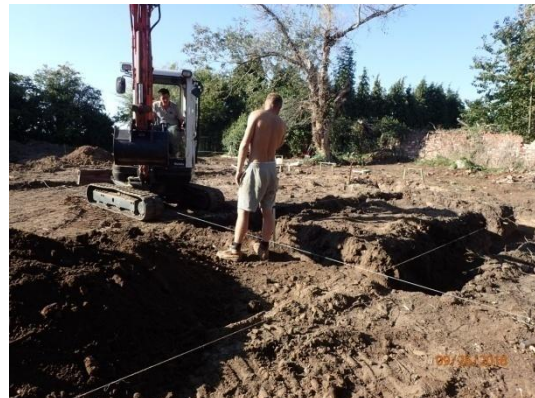
Plate 28: Excavation of the foundations, from the south-east
