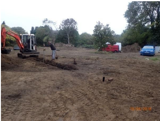
Plate 61: Excavation of the foundations, from the south
