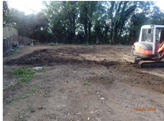
Plate 75: Excavation of the foundations, from the east
