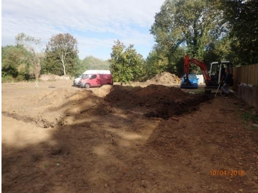
Plate 71: Excavation of the foundations, from the west
