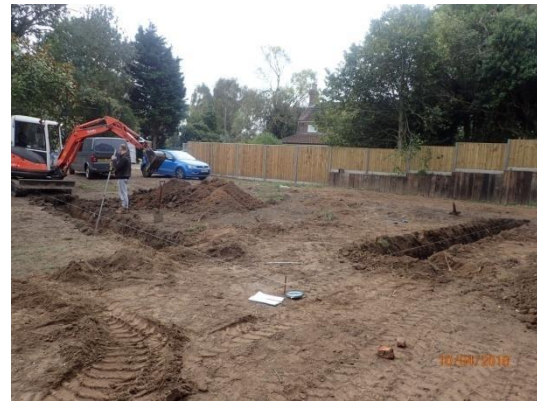
Plate 64: Excavation of the foundations, from the north-east
