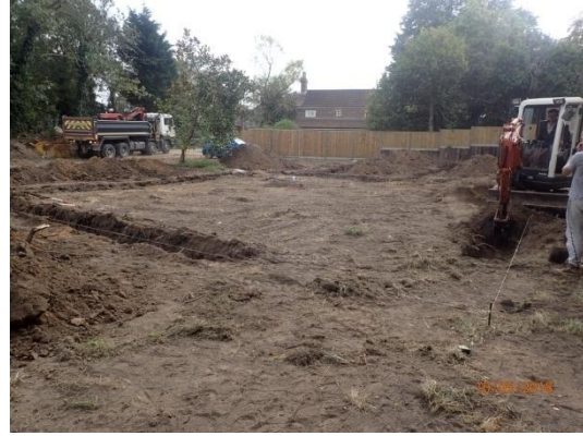
Plate 92: Excavation of the foundations, from the north-west
