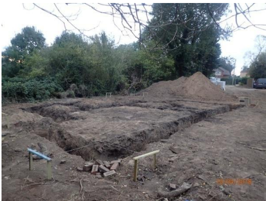
Plate 30: Completed foundation excavations, from the north-west
