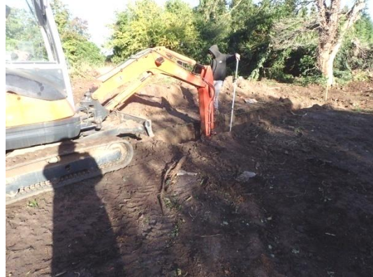
Plate 4: Excavation of the foundations, from the south
