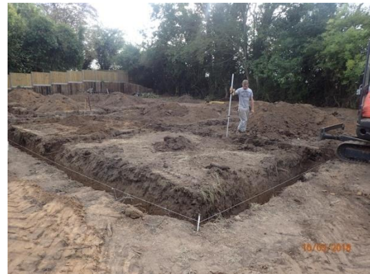
Plate 105: Excavation of the foundations, from the north-east
