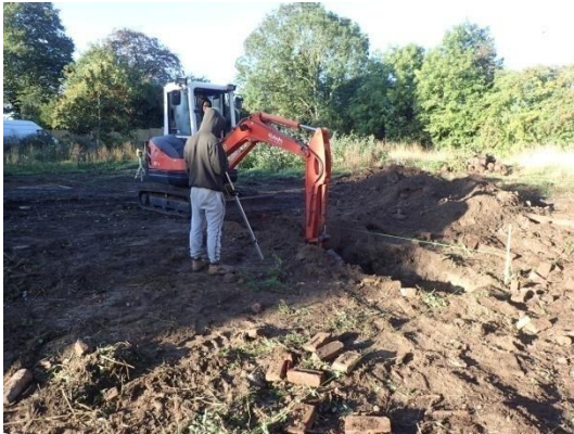
Plate 2: Excavation of the foundations, from the north-east
