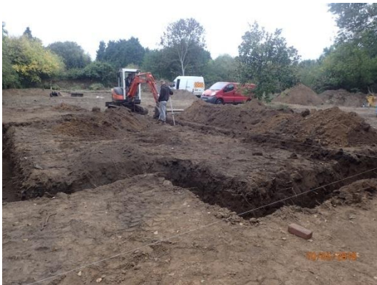
Plate 84: Excavation of the foundations, from the south-west
