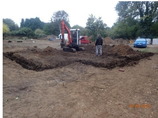
Plate 81: Excavation of the foundations, from the south-west
