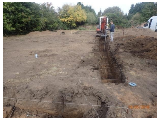
Plate 88: Excavation of the foundations, from the south
