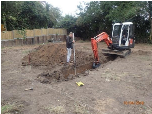
Plate 66: Excavation of the foundations, from the north-east
