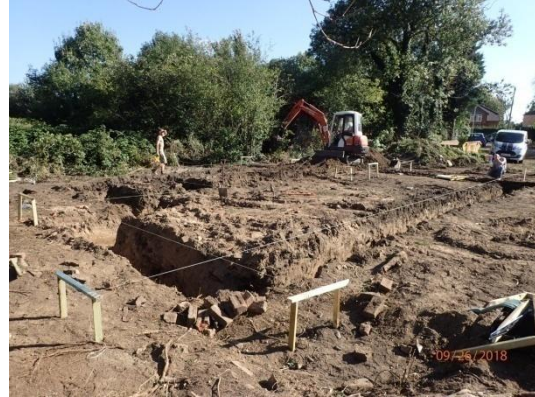
Plate 26: Excavation of the foundations, from the north-west
