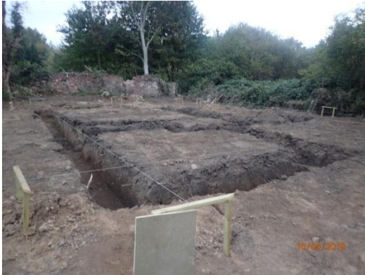
Plate 29: Completed foundation excavations, from the south
