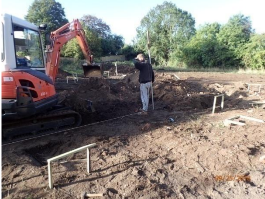
Plate 17: Excavation of the foundations, from the north-east
