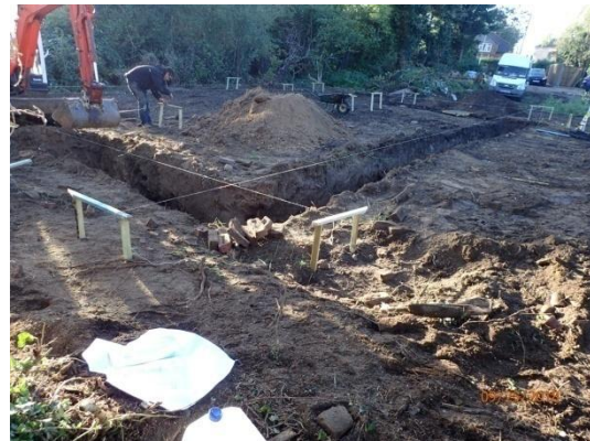
Plate 15: Excavation of the foundations, from the north-west
