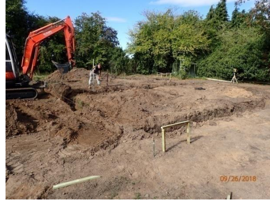
Plate 56: Excavation of the foundations, from the east
