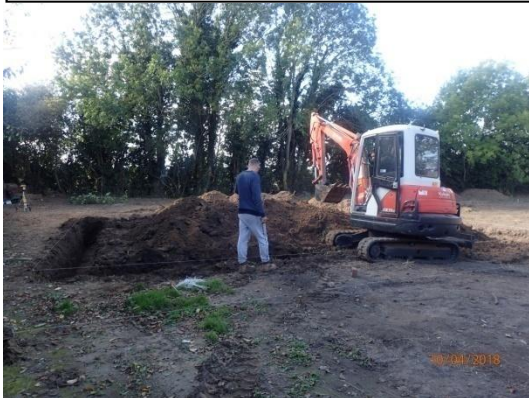
Plate 72: Excavation of the foundations, from the south
