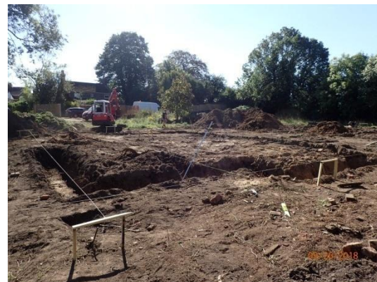
Plate 22: Excavation of the foundations, from the north-east
