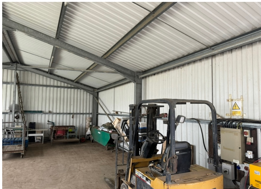
Figure 1: The internal structure of the building, showing the construction using steel frames and cladding.
