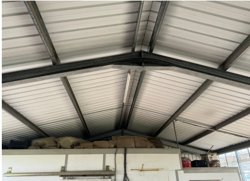
Figure 2: The ridge haunch of a portal frame in the building.
