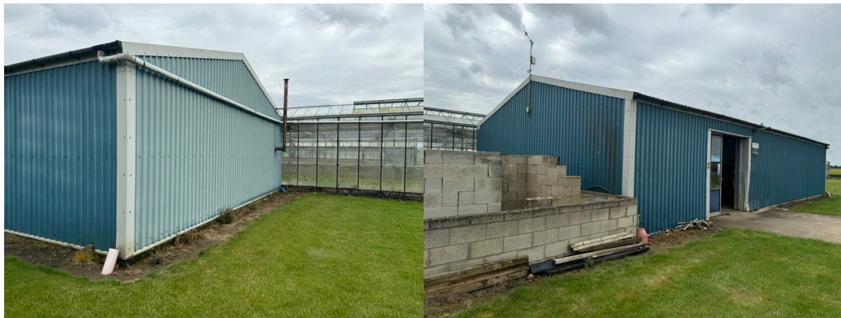
Figure 5 and 6: The exterior of the building
