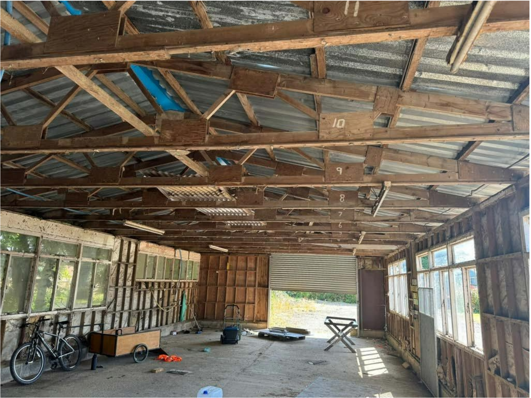
Image 4.0: View of timber trusses forming roof structure
