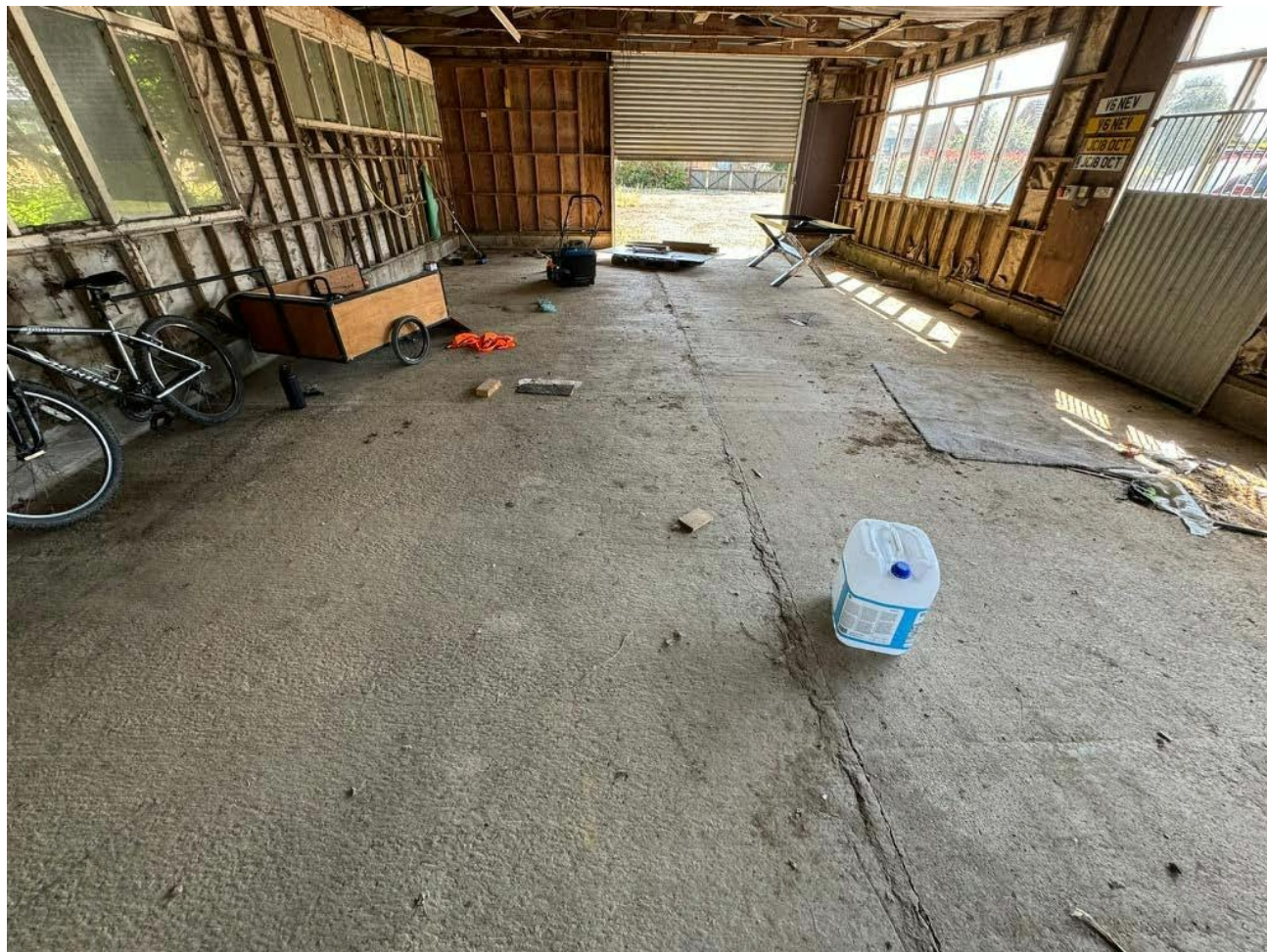
Image 1.0: View of concrete floor slab
