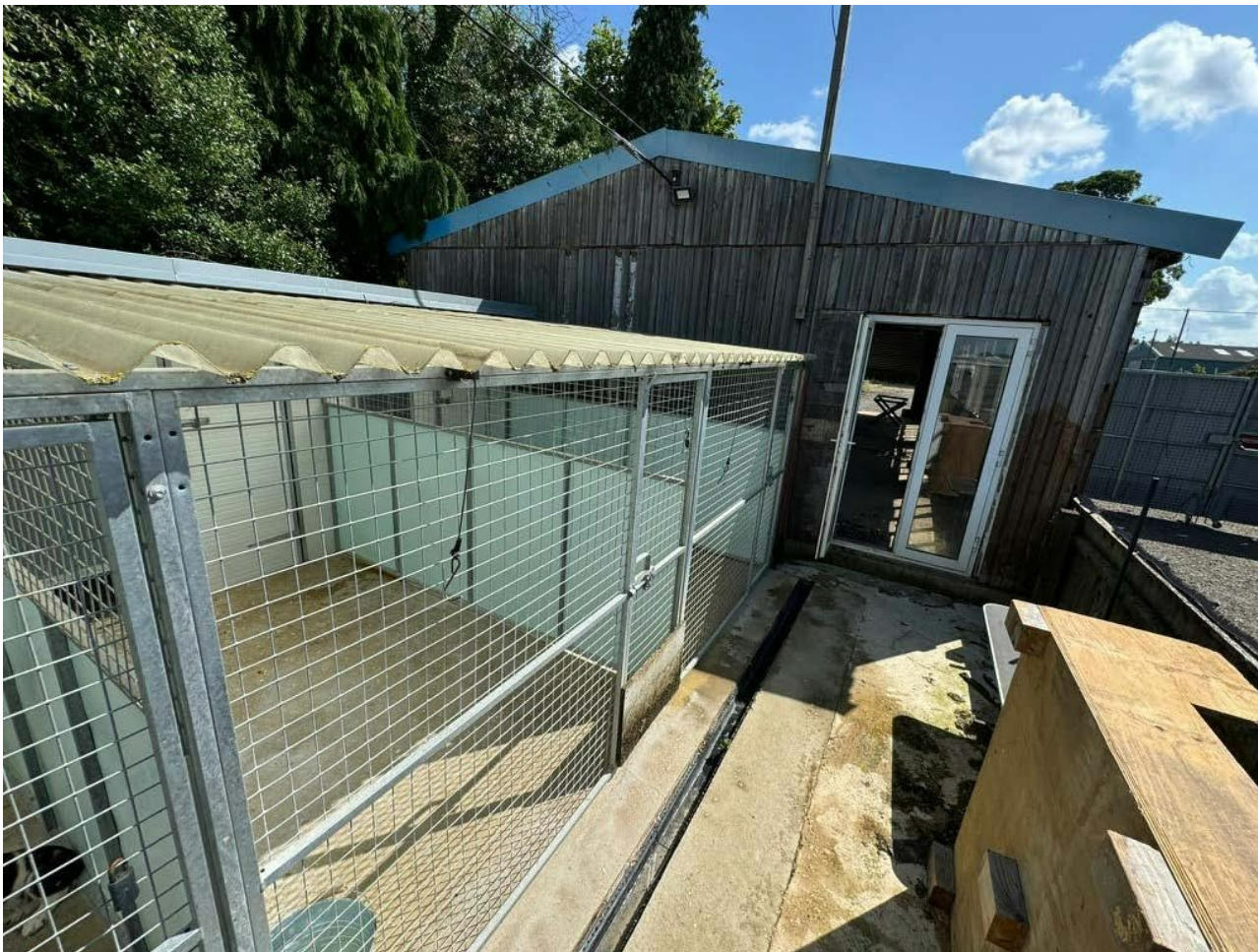
Image 8.0: View to rear of structure
