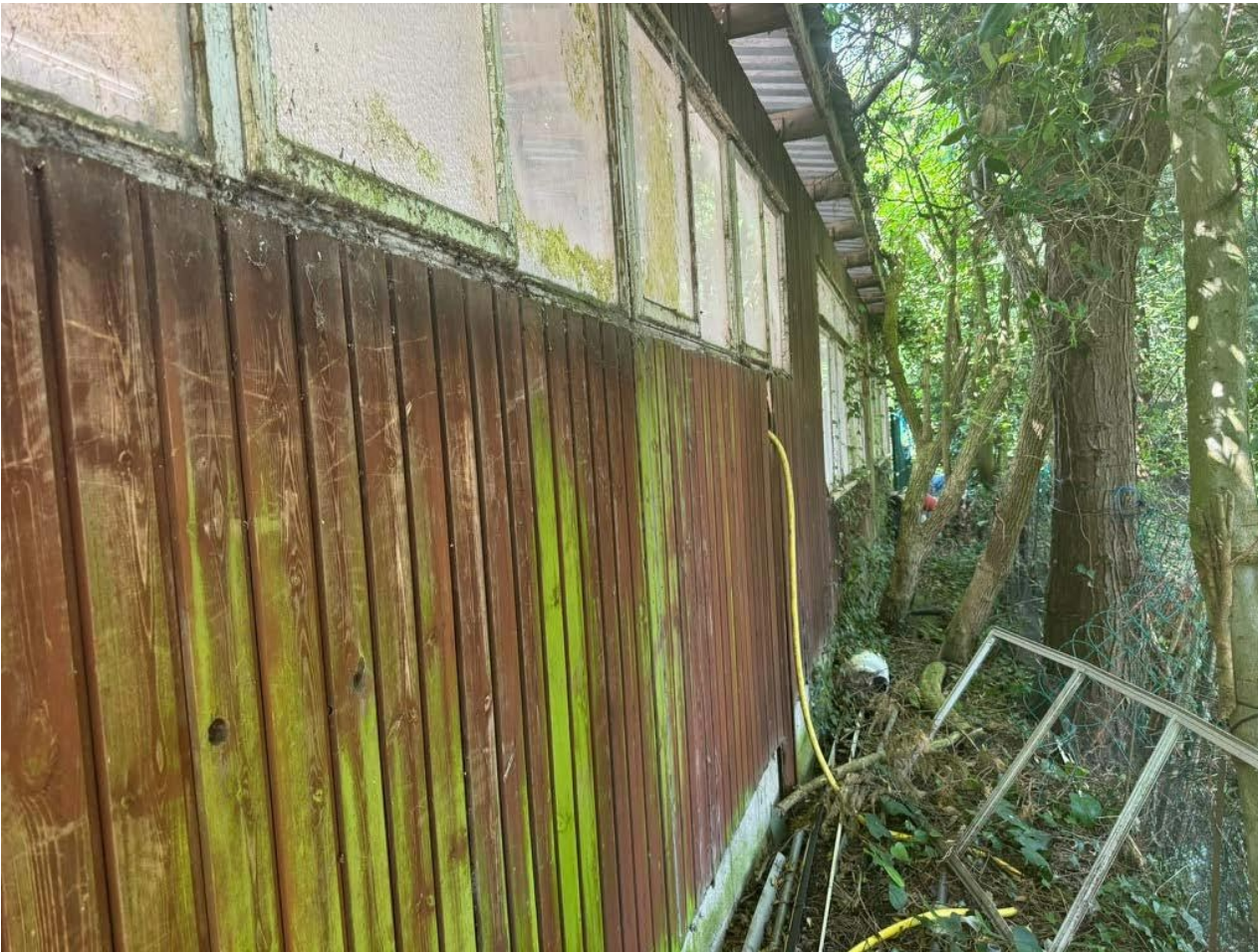
Image 7.0: View along opposite side elevation of structure
