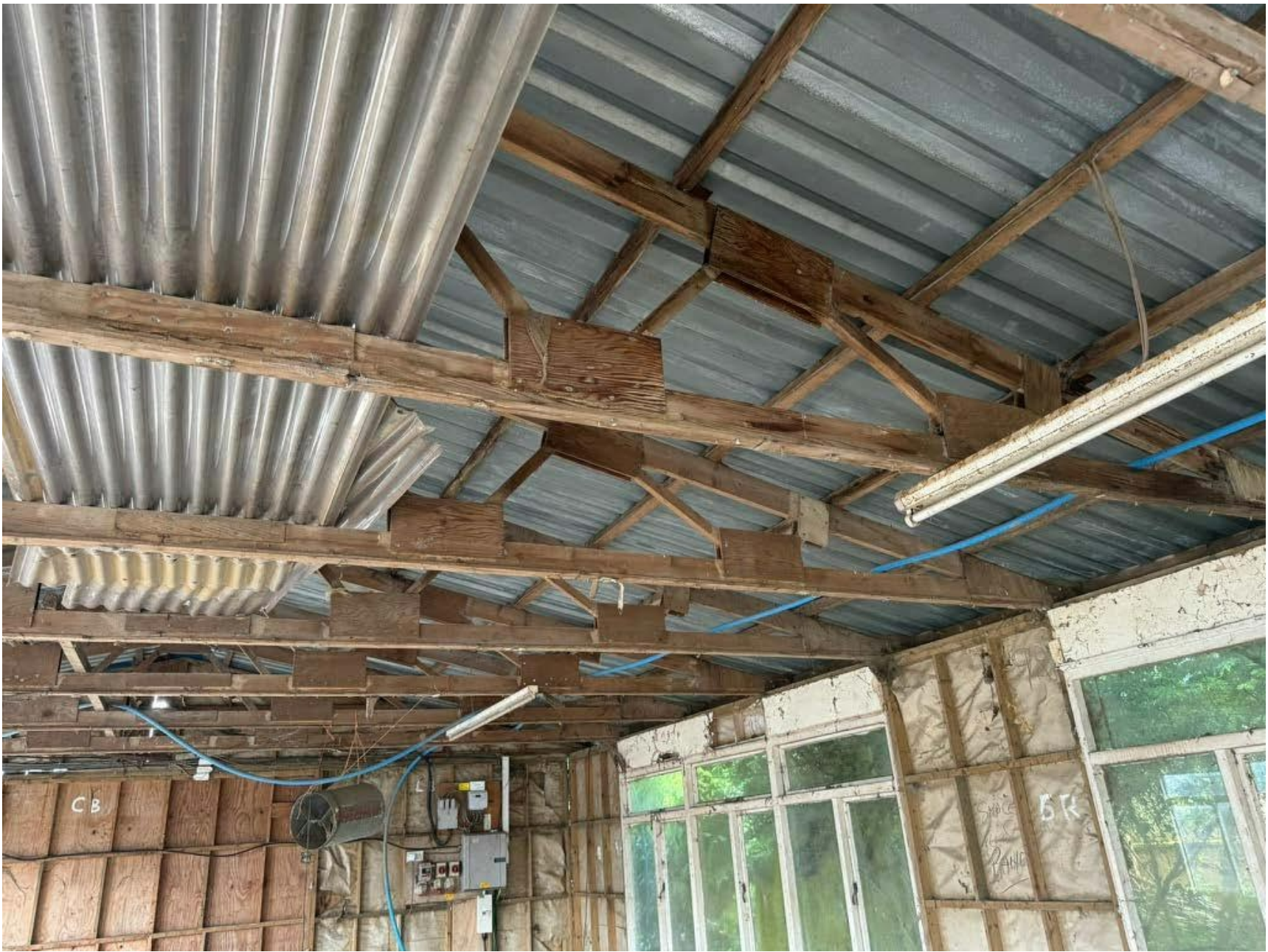
Image 5.0: View of corrugated steel roofing sheets
