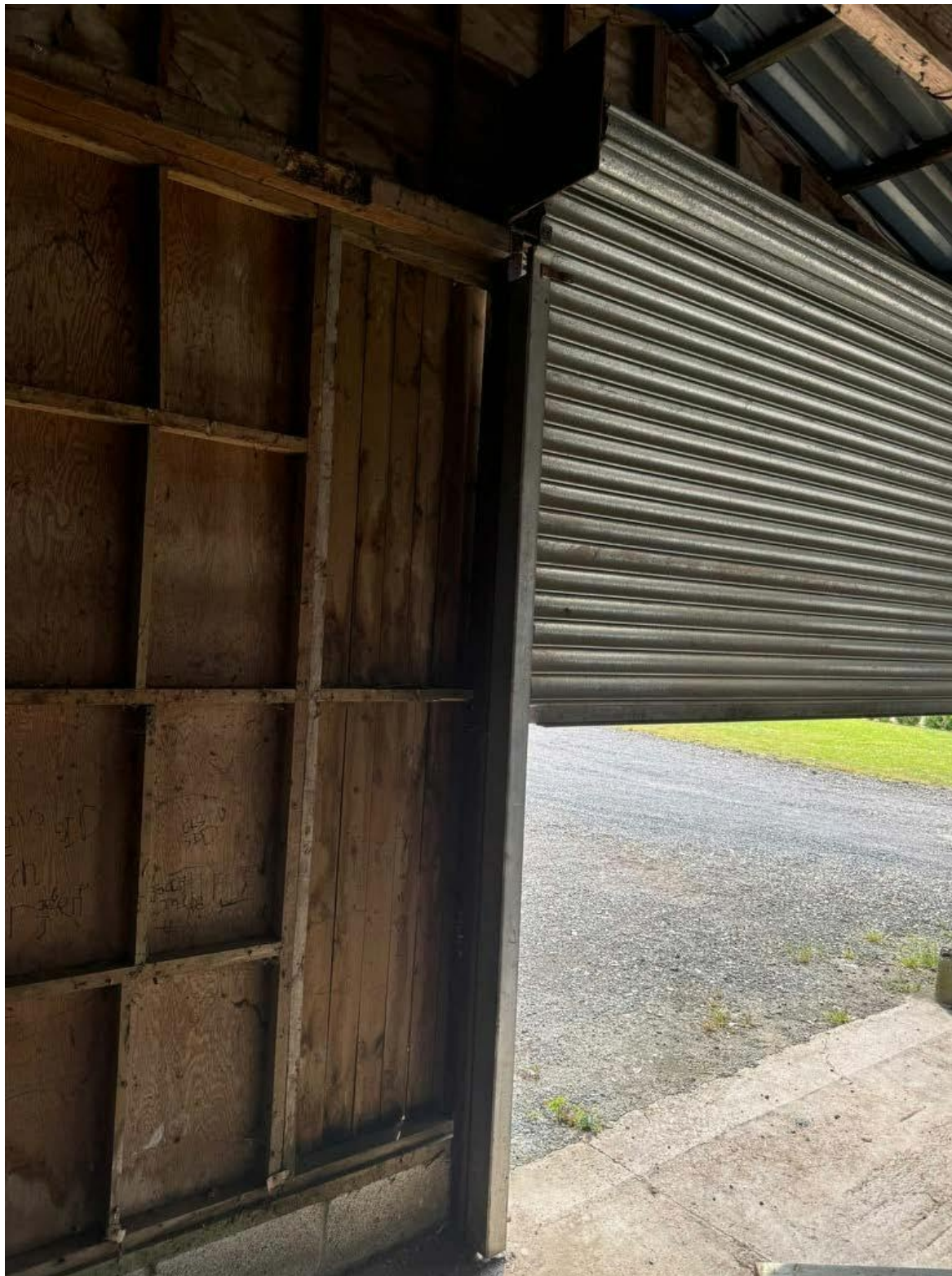
Image 6.0: View of steel support structure to front roller shutter door
