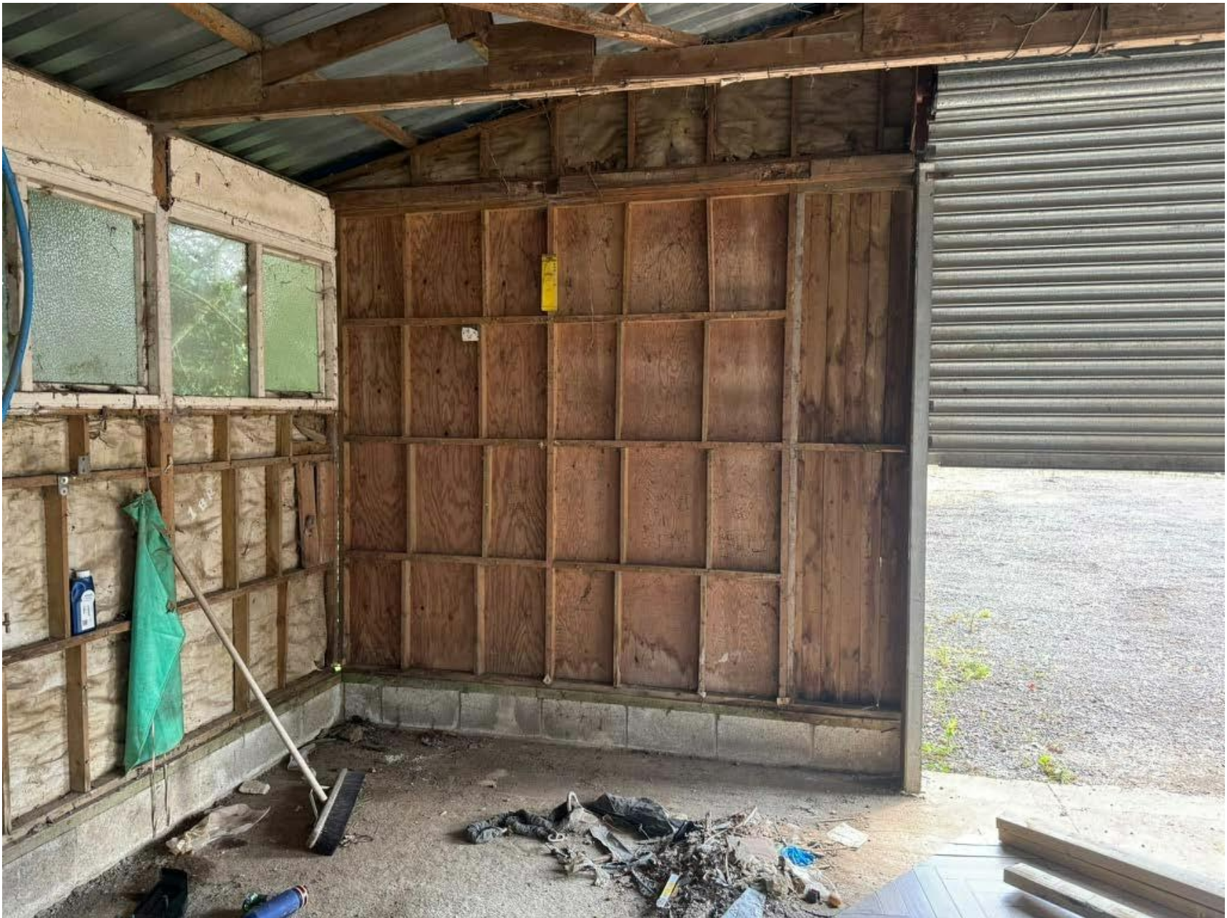
Image 3.0: Typical timber stud wall panel.
