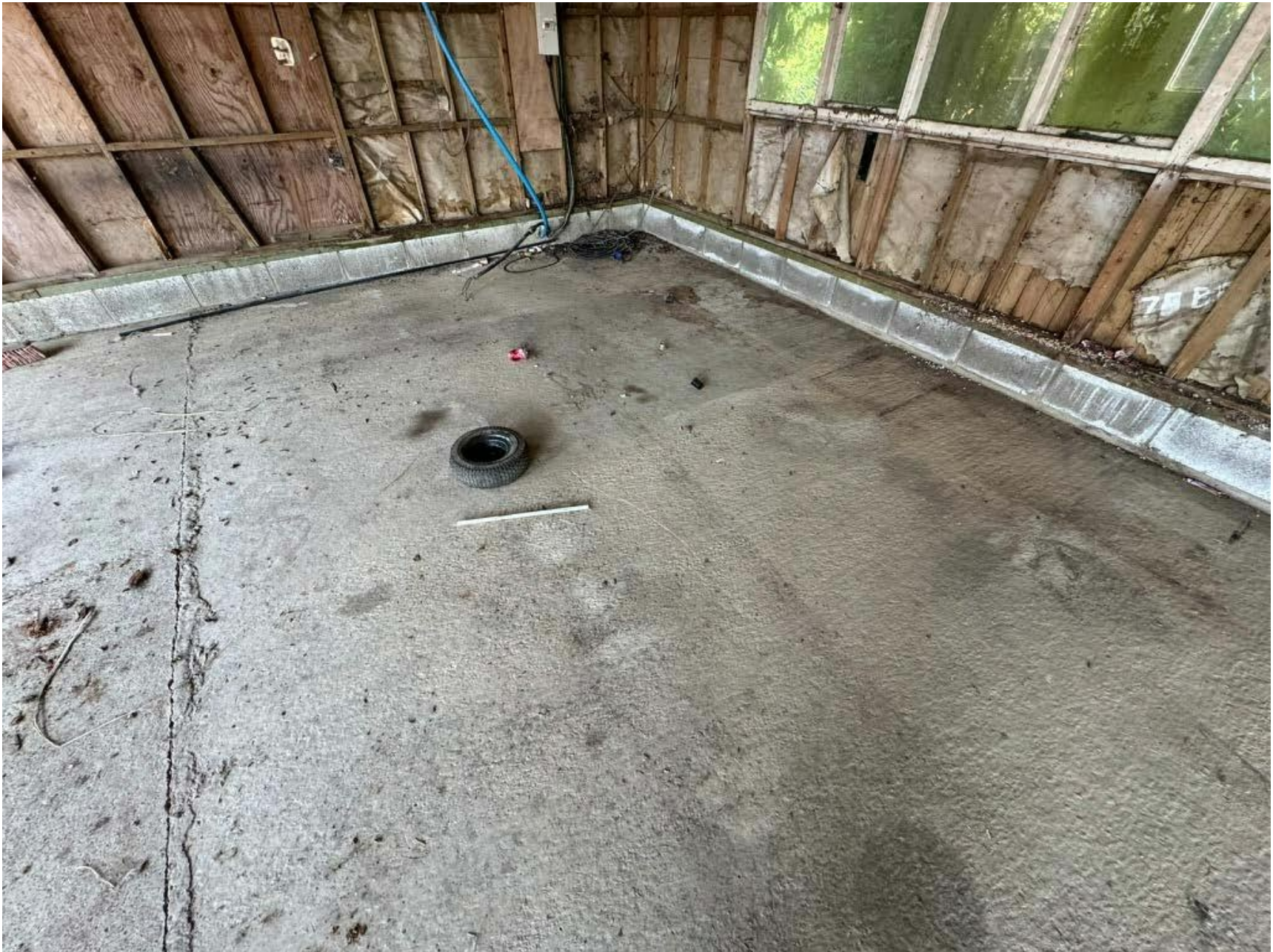
Image 2.0: drain holes to base of structure.
