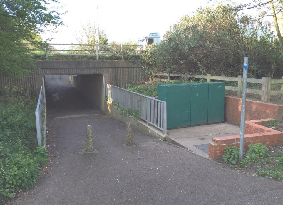
Pedestrian and cycle underpass to the A17
