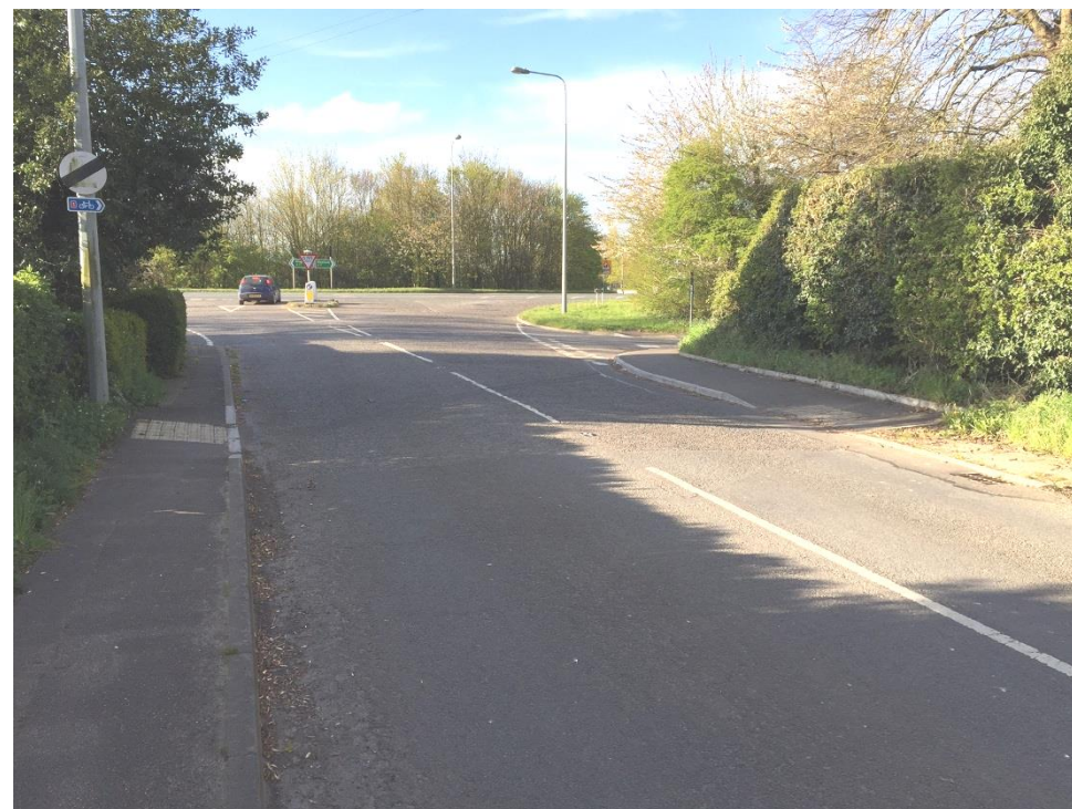
Footpath improvements to Penny Hill Road undertaken under Planning Approval H09-0789-11
