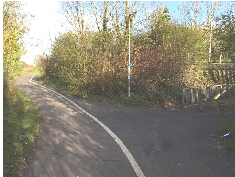
A17 Underpass & footpath/ cycleway
