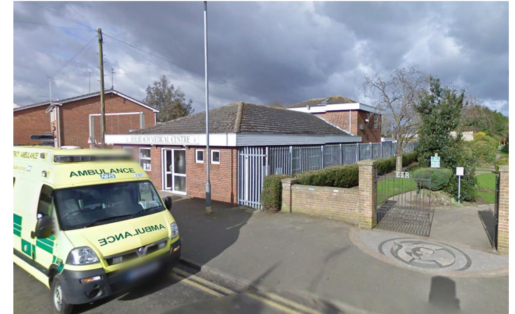
Monroe Medical Centre, Park Road
