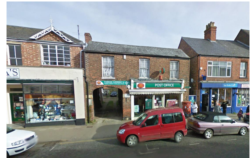
Post Office along the High Street
