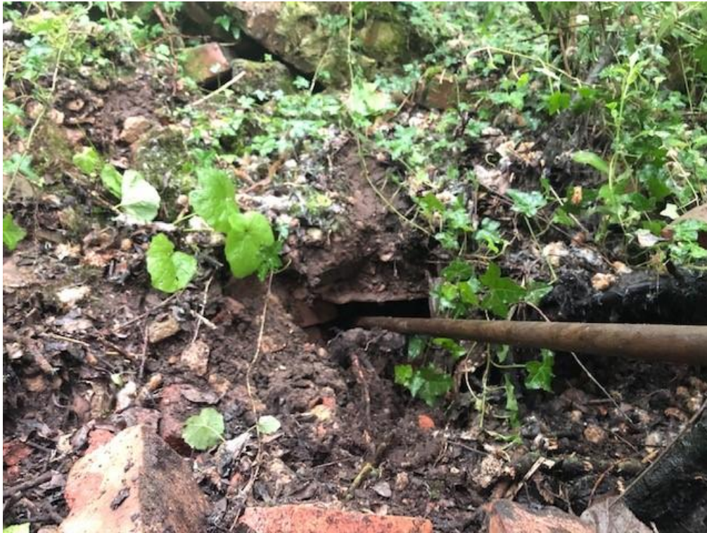
Image 2: Image of Pipe termination point.
