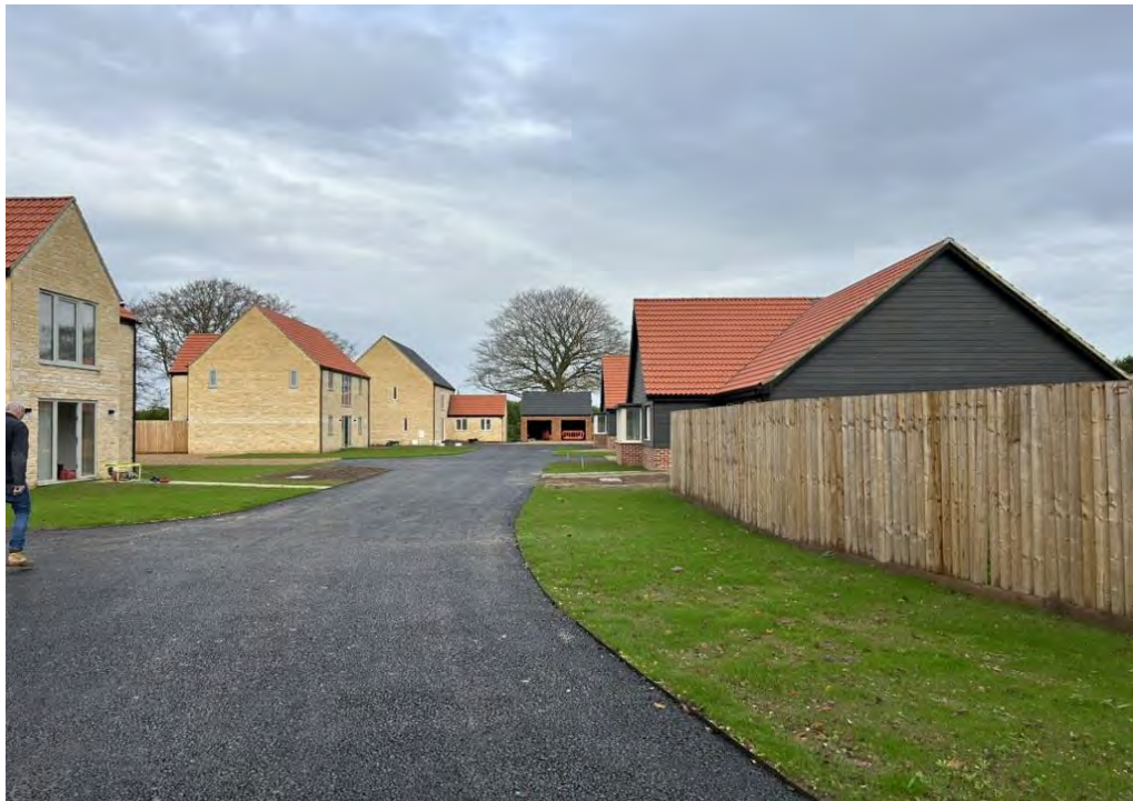
Photograph 4: On site buildings and hardstanding
