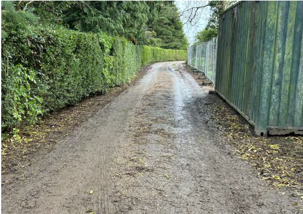
Photograph 3: Access track to the site
