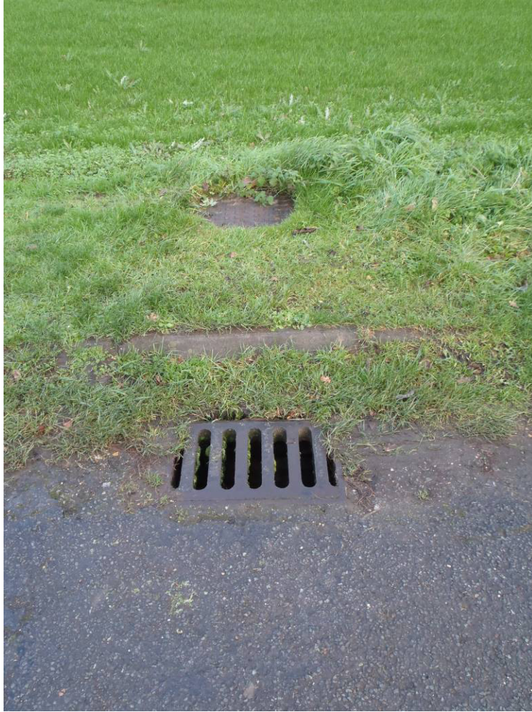
Plate 4 – Manhole cover and drain on the edge of the Site, looking north
