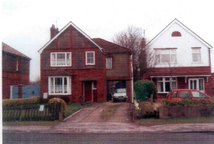
House showing new extension
