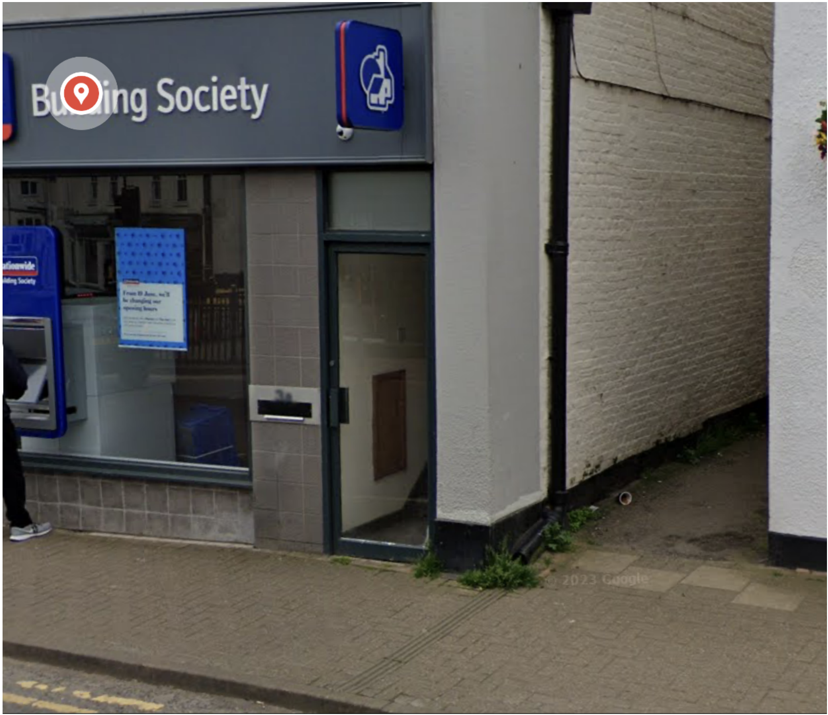
IMAGE OF SIDE ELEVATION DEFIBRILLATOR AND BLEED KIT ARE FIXED TO
