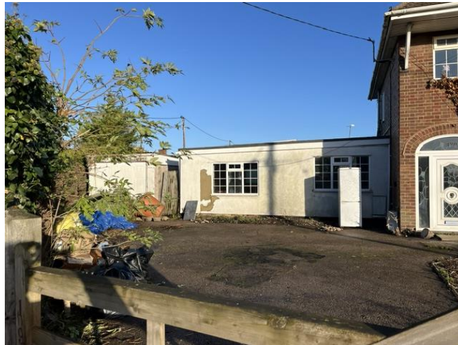
Flat roofed extension as approved 1985
