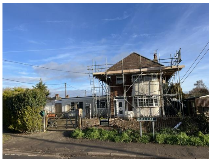
No.190 Hallgate undergoing refurbishment
