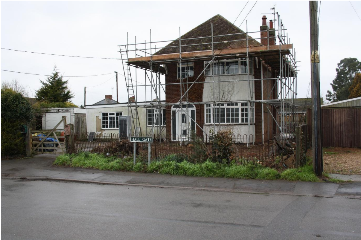
View of site from Hallgate
