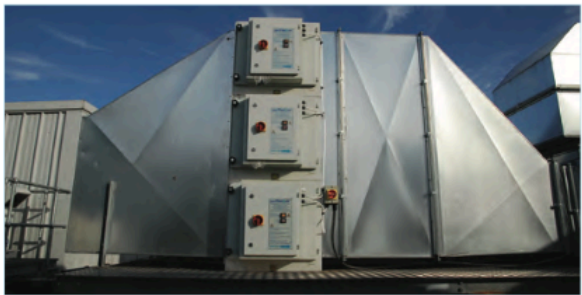
3 ESP Units Stacked in modular formation
