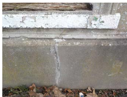
Photo 6 – Previously repointed cracking below ground floor window
