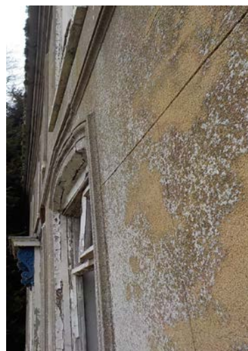
Photo 6 – Previously repointed cracking below ground floor window
