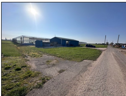
Figure 4 – Concrete hardstanding and buildings
