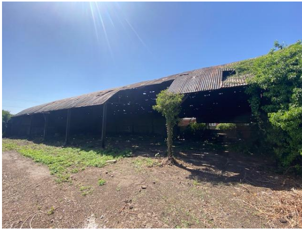
East elevation of agricultural building and internals showing decayed structure.
