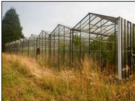
Photo 5 Western Elevation of glasshouse
