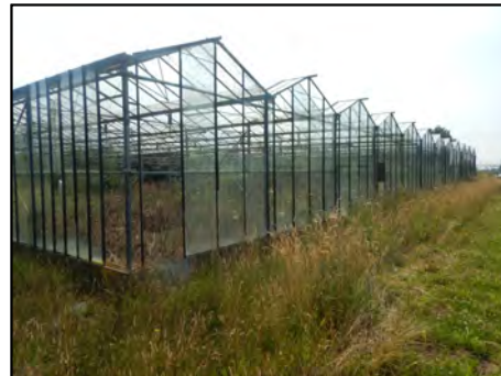
Photo 6 Western elevation of glasshouse
