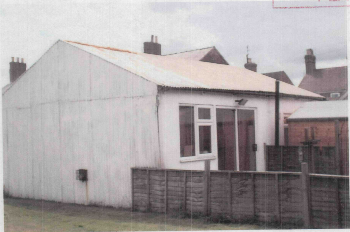
(west) Side and rear elevation of Annexe
