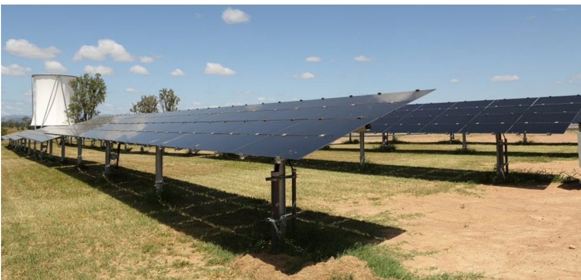
Figure 2.6: Typical Single Axis Tracking Solar Arrays
