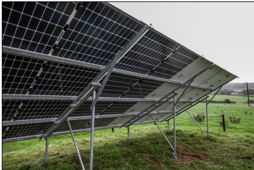
Figure 2.4: Typical solar array with bi-facial solar panels
