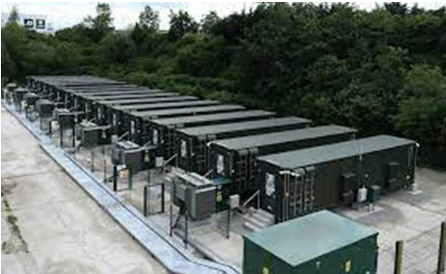
Figure 2.9: Typical Battery Storage Containers
