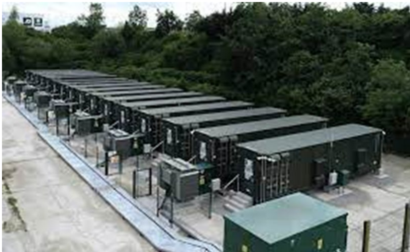
Figure 7 - Typical Battery Storage Containers
