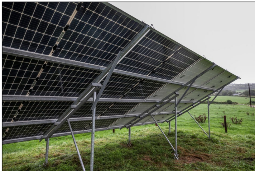
Figure 2 - Typical solar array with bi-facial solar panels
