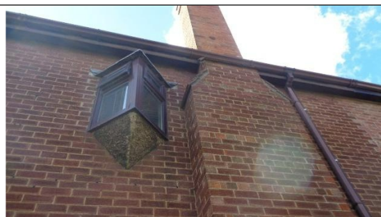
Photo 2: Typical soffit/ wall connection on house
