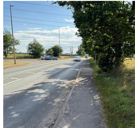
Plate 2: Photo of A151/Wignals Gate Junction
