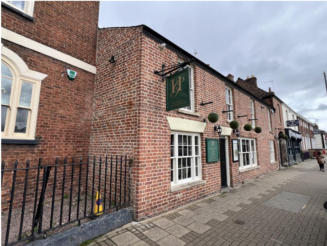
Fig 01. View of the High Street frontage from the south-west.
