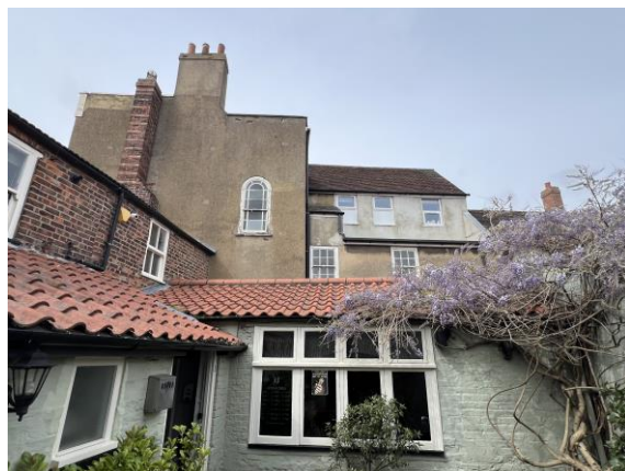
Fig 05. View west across the rear courtyard.
