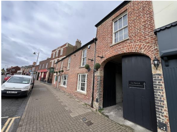
Fig 02. Carriage arch access from High Street.
