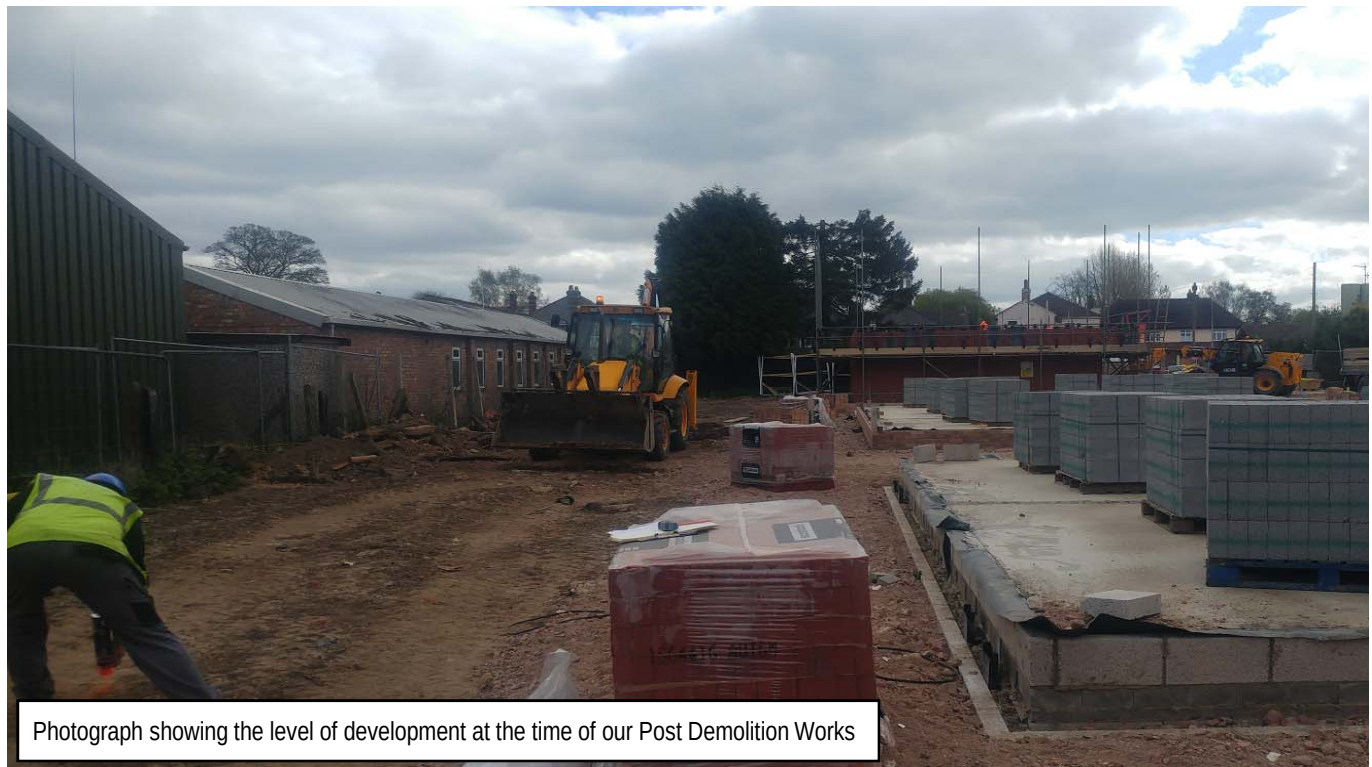
Photograph showing the level of development at the time of our Post Demolition Works
