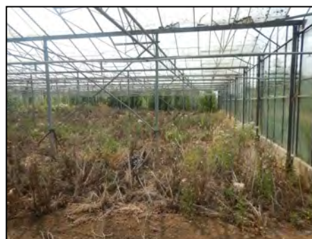
Photo 7 Interior of glasshouse
