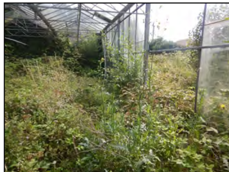
Photo 10 Interior of glasshouse
