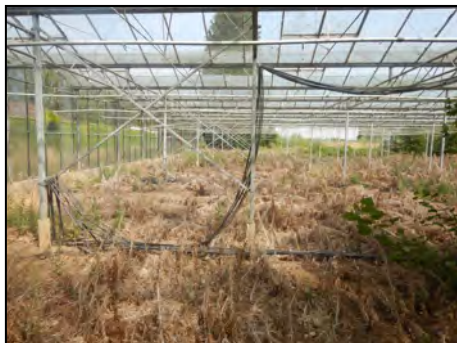
Photo 9 Interior of glasshouse
