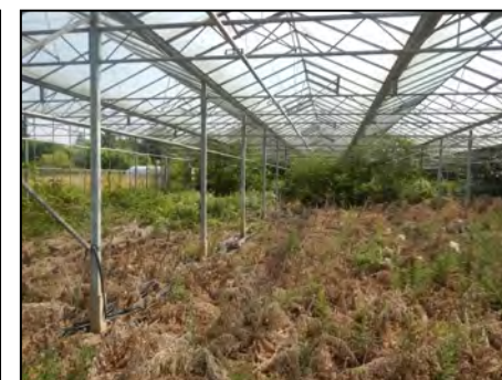
Photo 8 Interior of glasshouse
