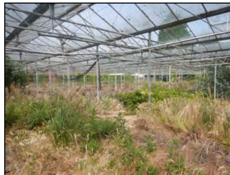
Photo 11 Interior of glasshouse
