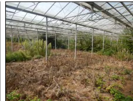
Photo 12 Interior of glasshouse
