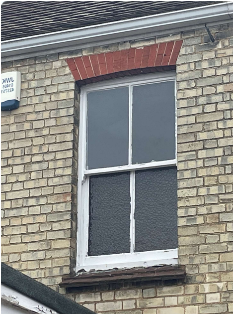
Window 2 – rear elevation
