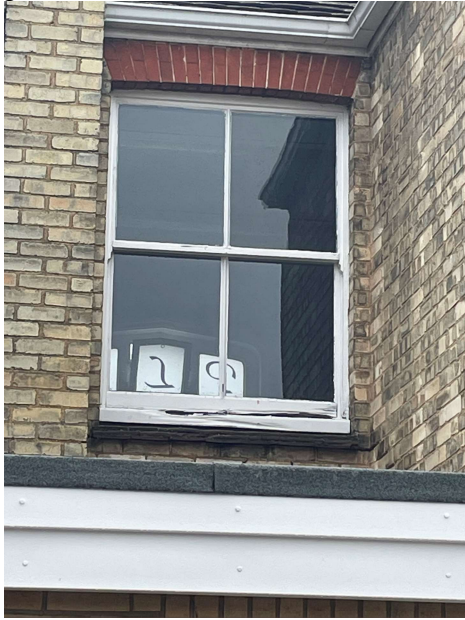
Window 1 – rear elevation
