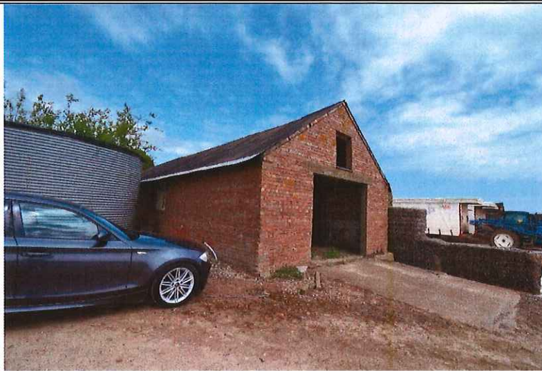
Image 2: Existing View of Barn 2
