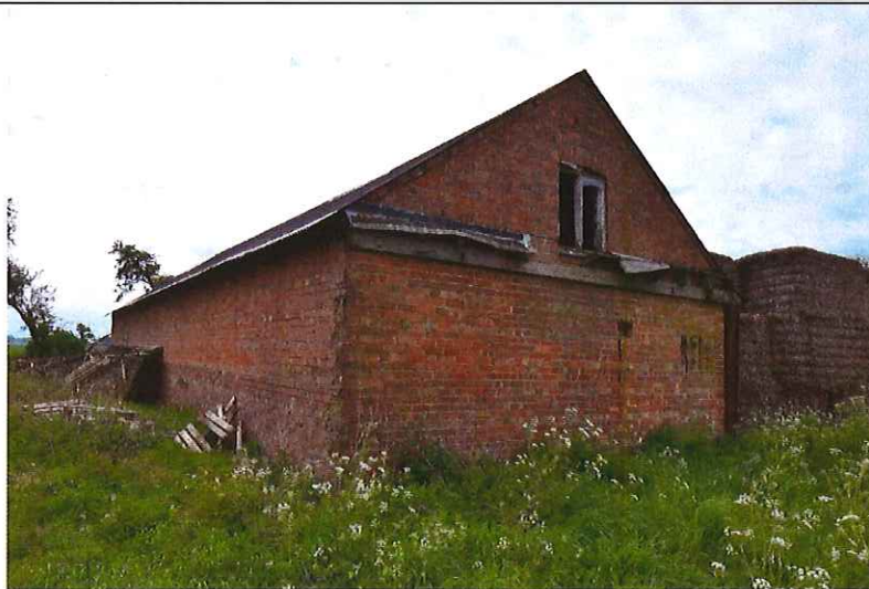
Image 1: Existing View of Barn 1
