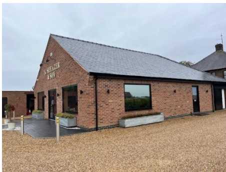
H09-0932-24 - Extension to Shop, completed late 2025
