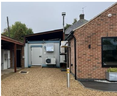
H09-0748-20 – Prefabricated Unit in situ
