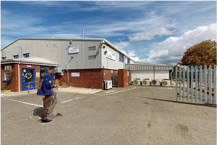
View looking East towards the Site.
