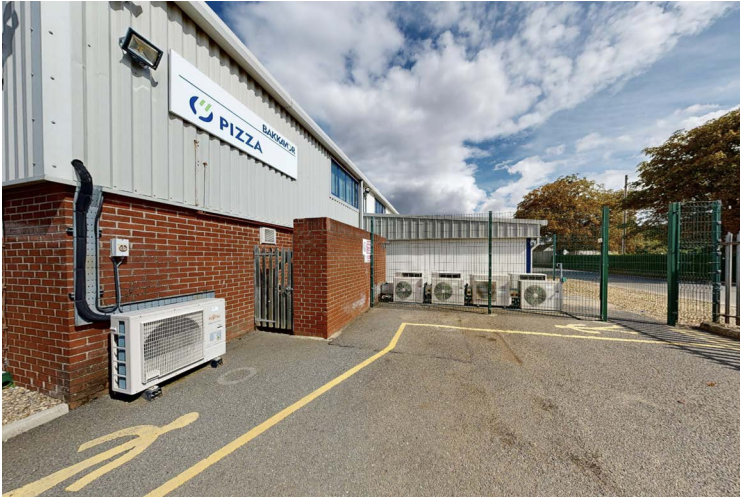
View looking East towards the Site.
