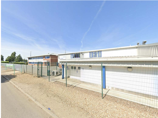
View looking North West towards the Site.
