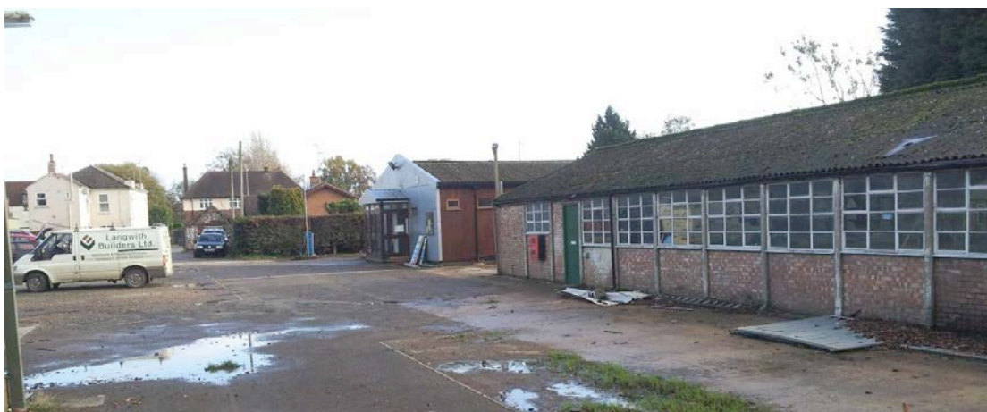
The whole yard area looks run down, and un-maintained and does not contribute to the 'visual amenity' of this area of Holbeach..
