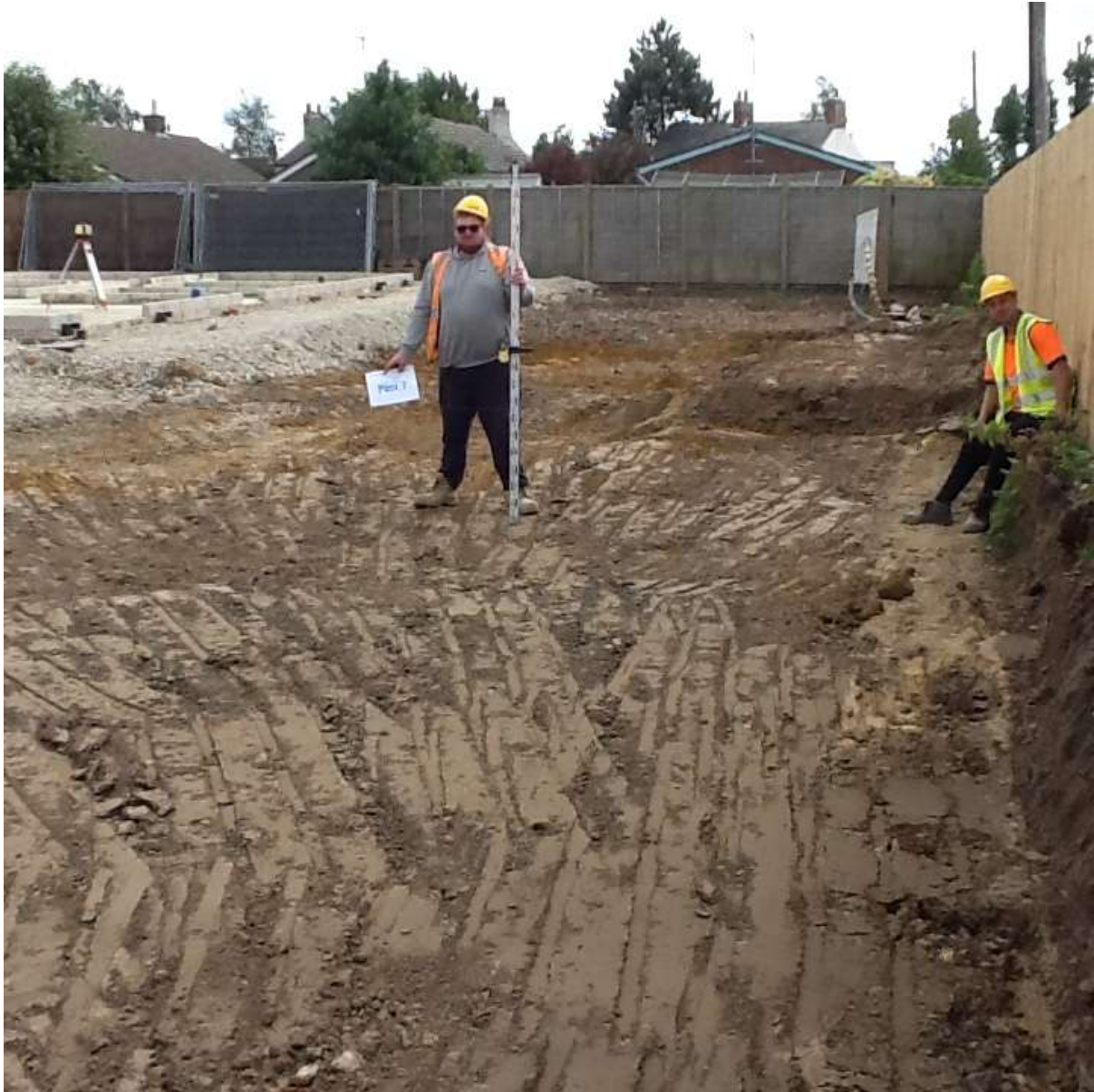
Photo 14 Rear garden of plot 7 showing area excavated
