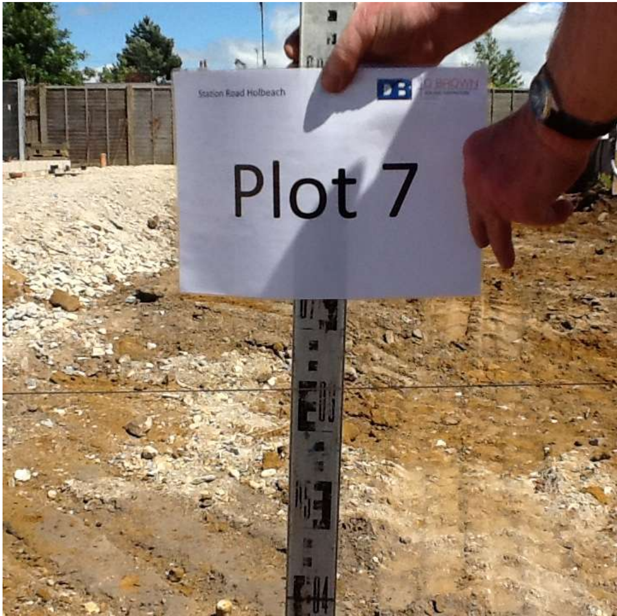
Photo 13 Rear garden of Plot 7 showing depth of excavation
