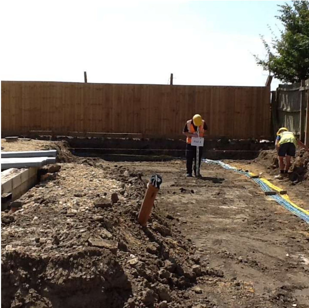
Photo 8 Rear garden of plot 4 showing area excavated
