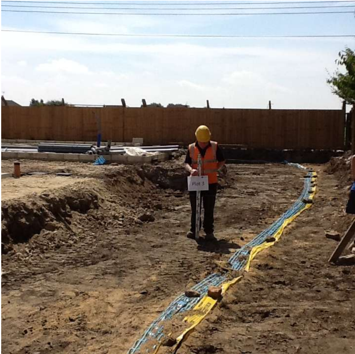
Photo 6 Rear garden of plot 3 showing area excavated
