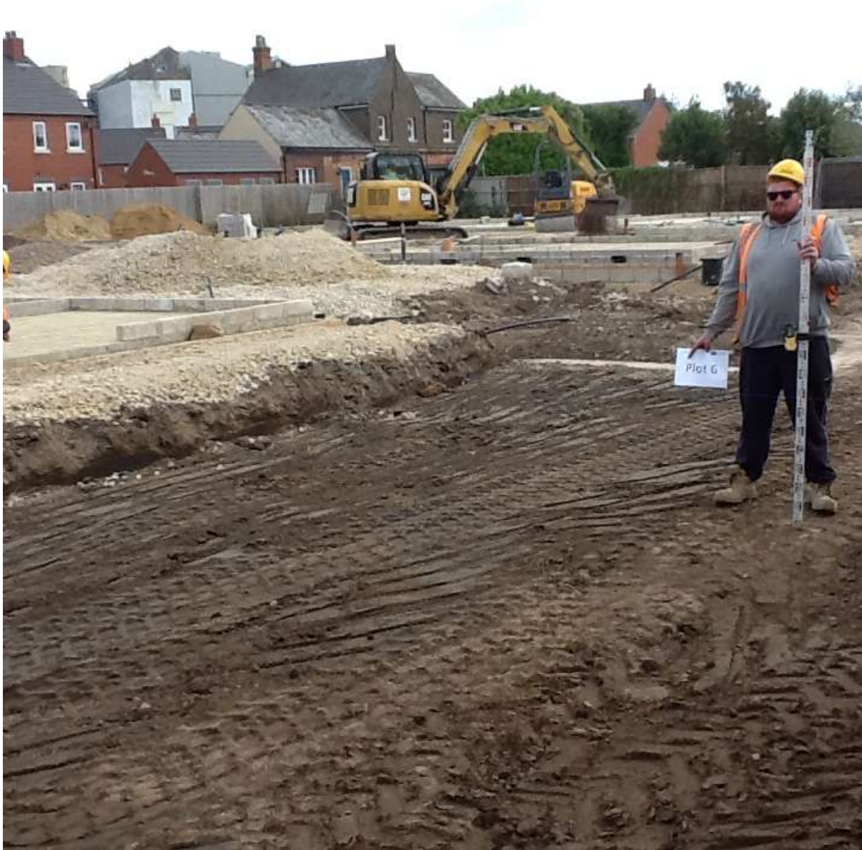
Photo 12 Rear garden of plot 6 showing area excavated
