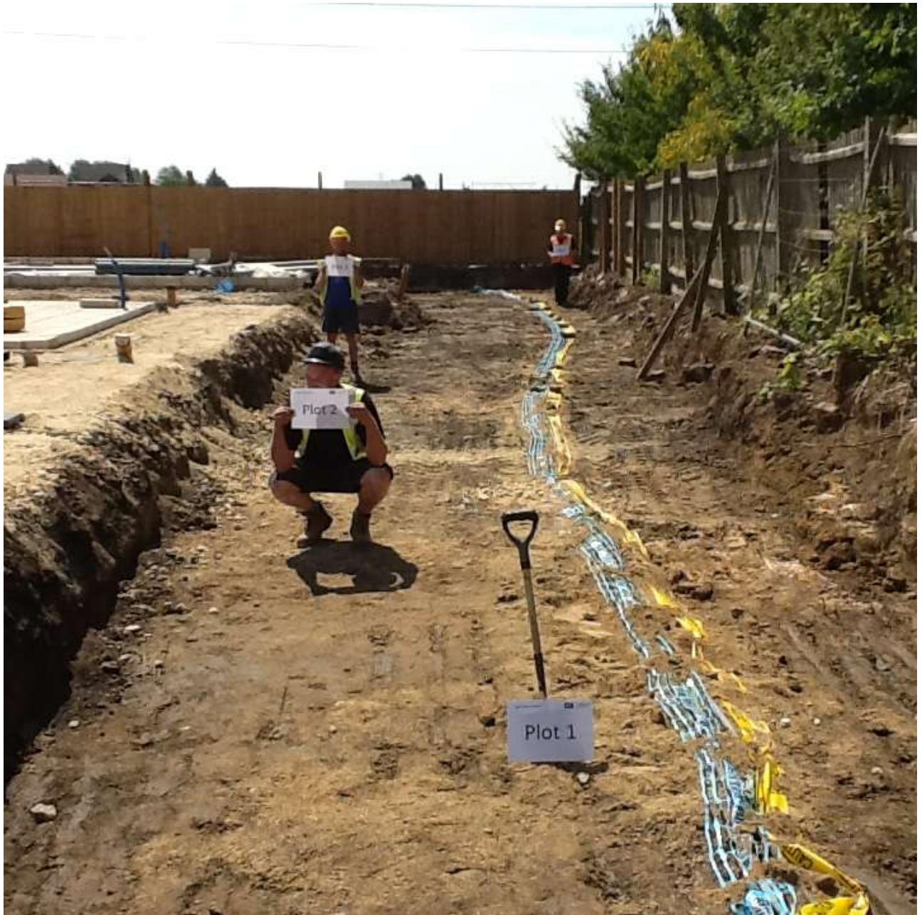
Photo 2 Rear garden of plot 1 showing area excavated
