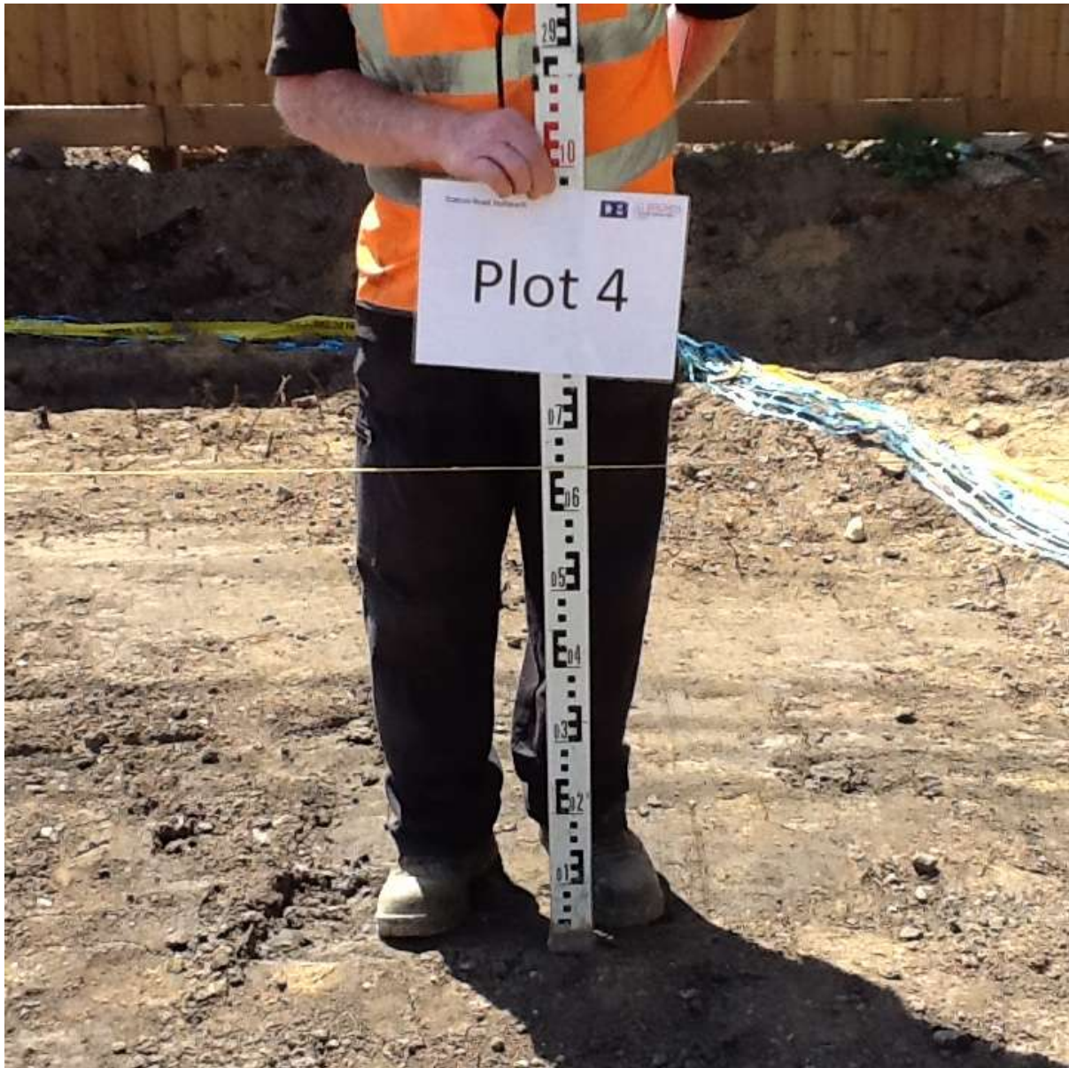
Photo 7 Rear garden of Plot 4 showing depth of excavation
