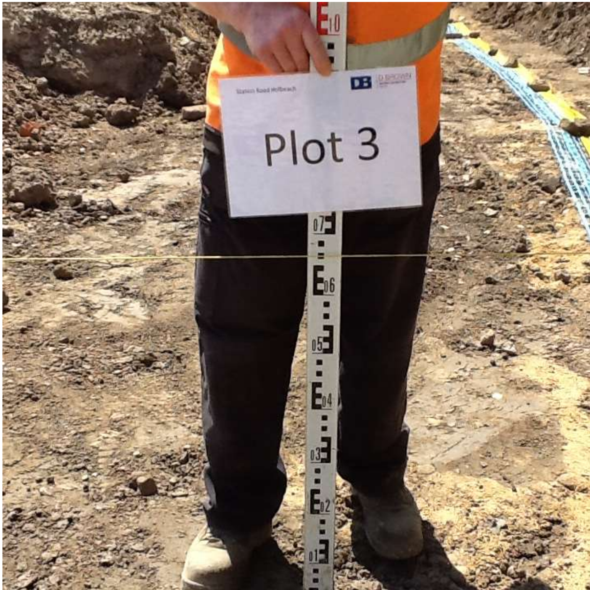
Photo 5 Rear garden of Plot 3 showing depth of excavation
