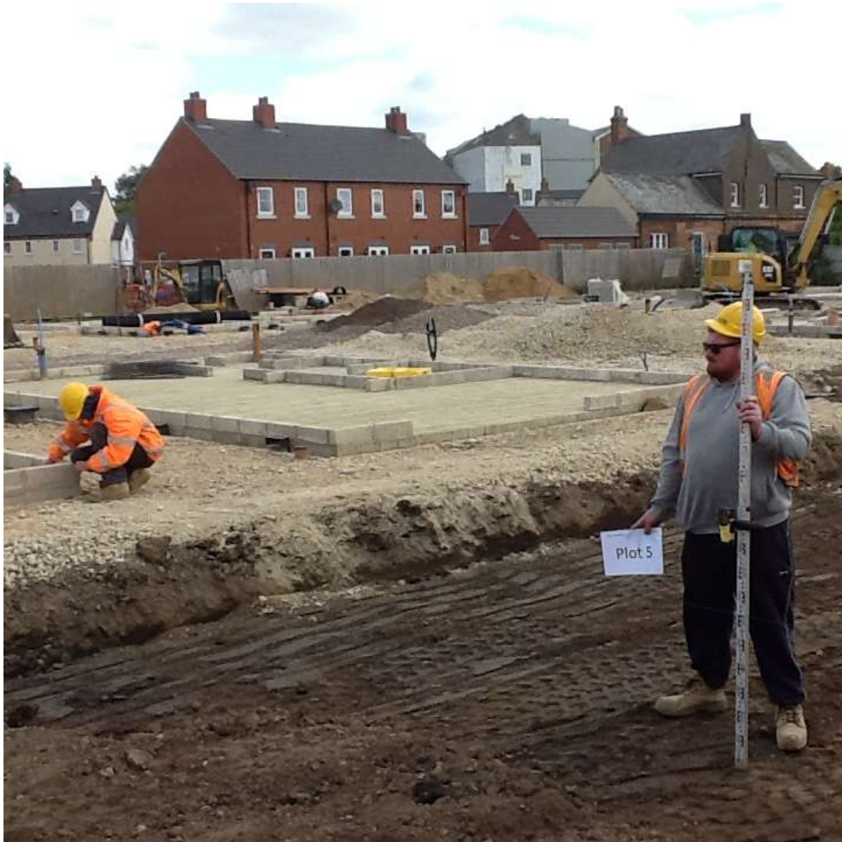
Photo 10 Rear garden of plot 5 showing area excavated
