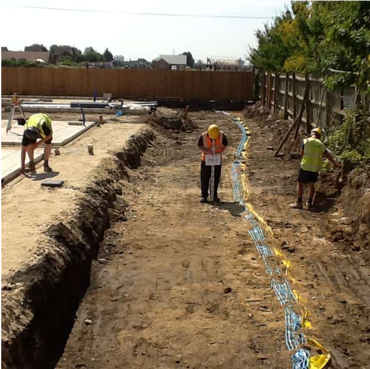
Photo 4 Rear garden of plot 2 showing area excavated
