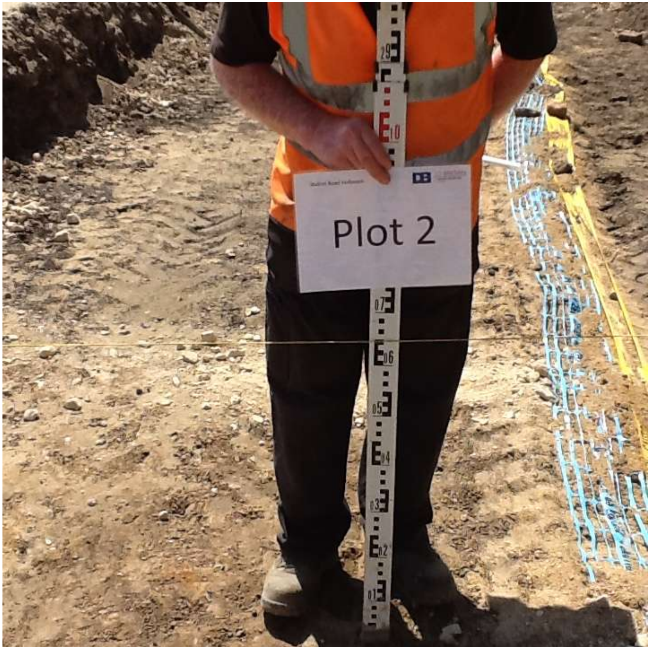
Photo 3 Rear garden of Plot 2 showing depth of excavation
