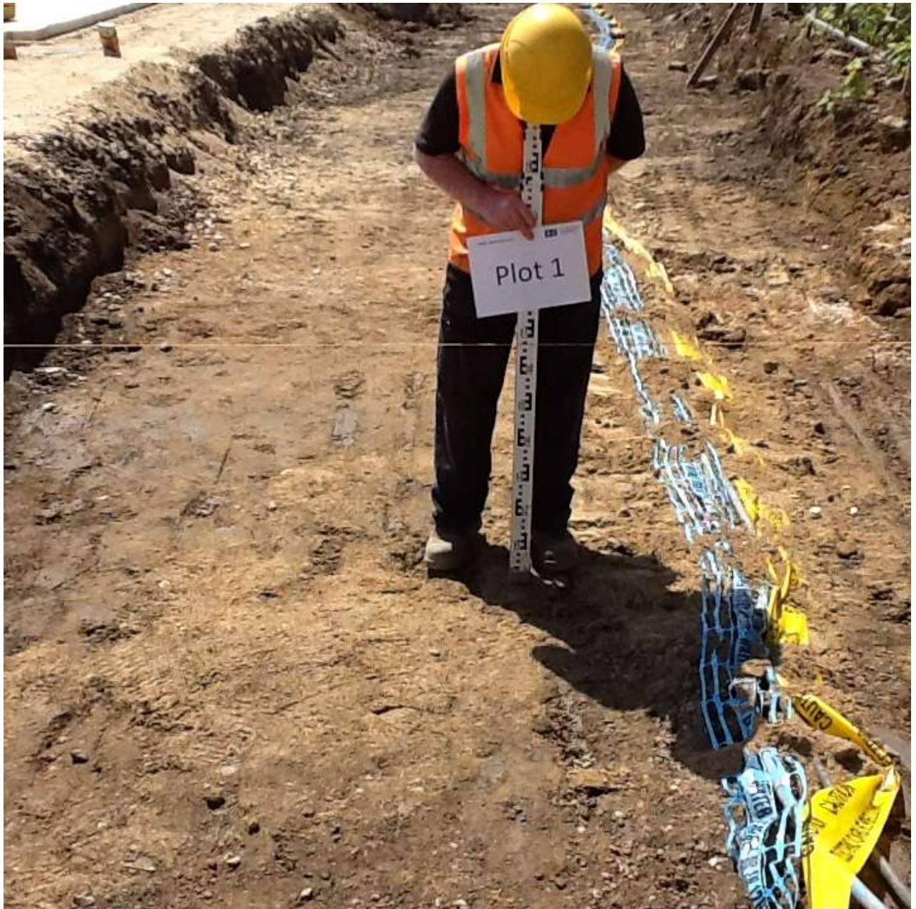
Photo 1 Rear garden of plot 1 showing depth of excavation
