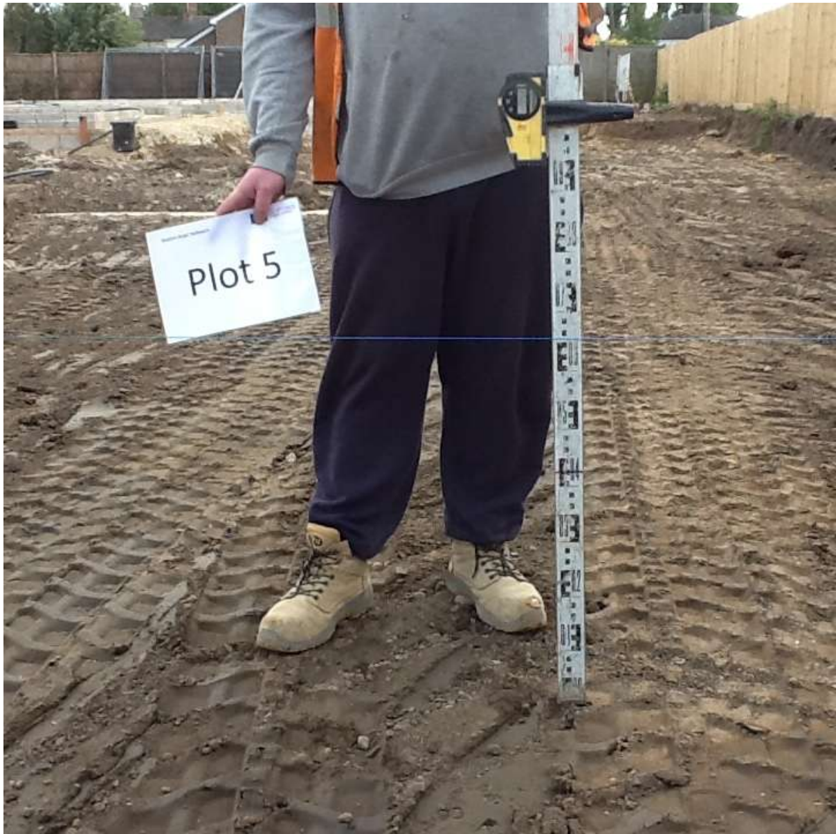
Photo 9 Rear garden of Plot 5 showing depth of excavation
