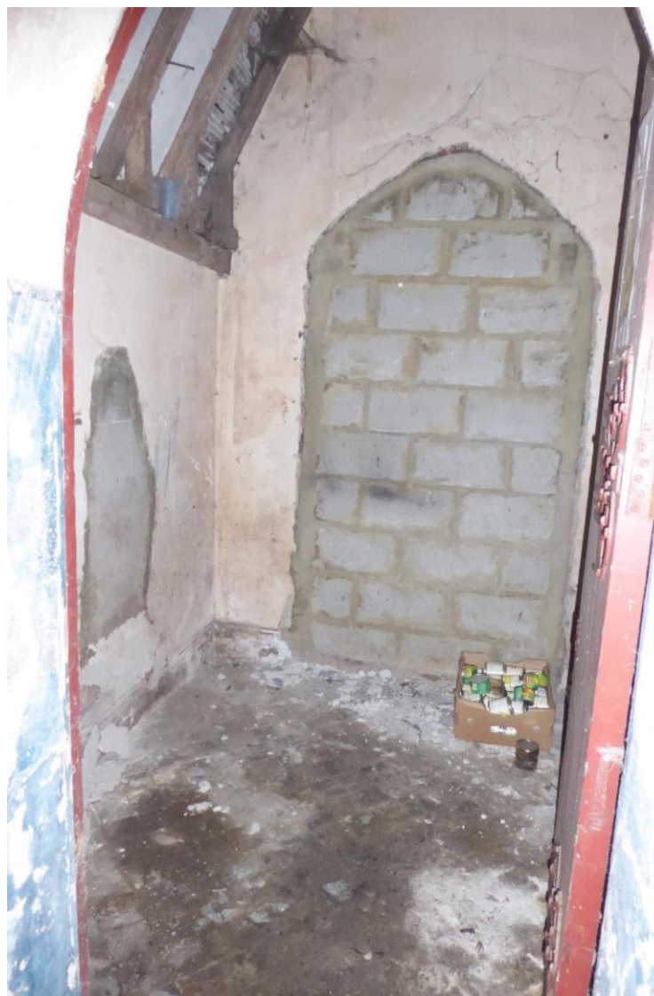
North vestry interior looking north
