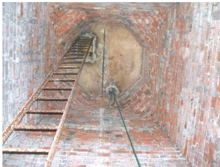
Tower room above carriage porch, view upwards
