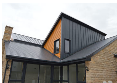
Example of zinc wall cladding
