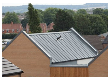
Example of zinc roofing
