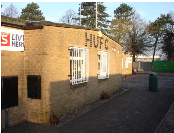
Existing front of building
