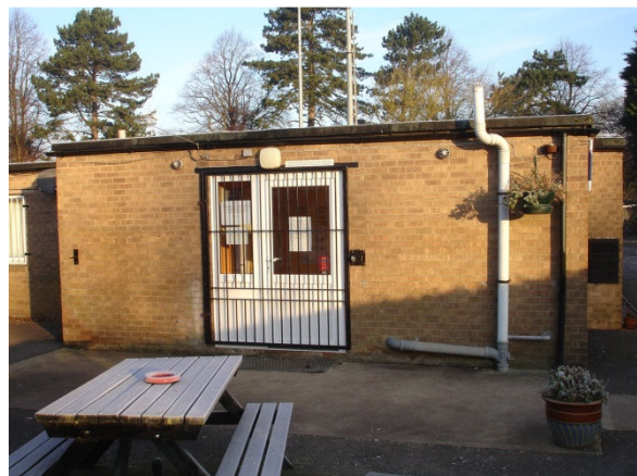
Existing main entrance
