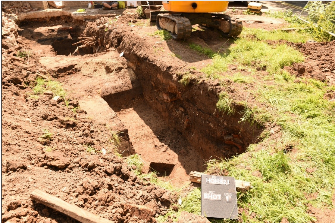
Plate 5: Looking south with Section 1 to right.
