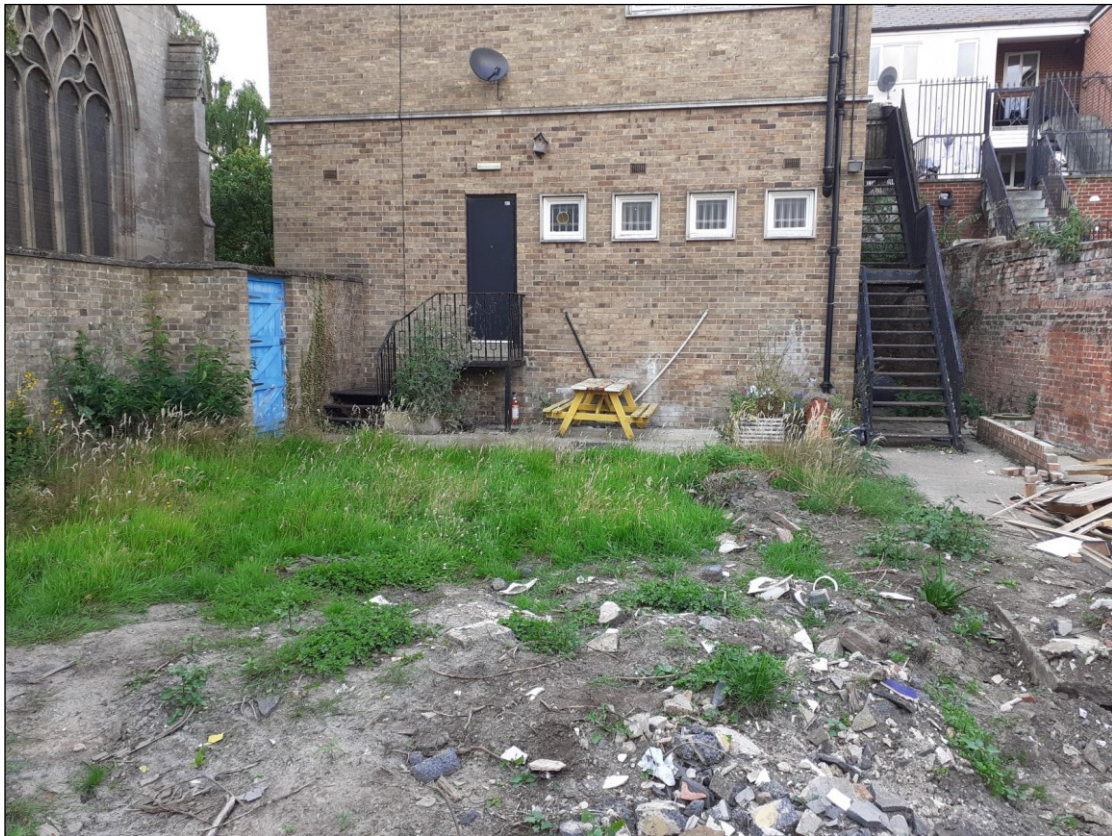
Plate 2: Northern The site prior to trial trenching, looking north
