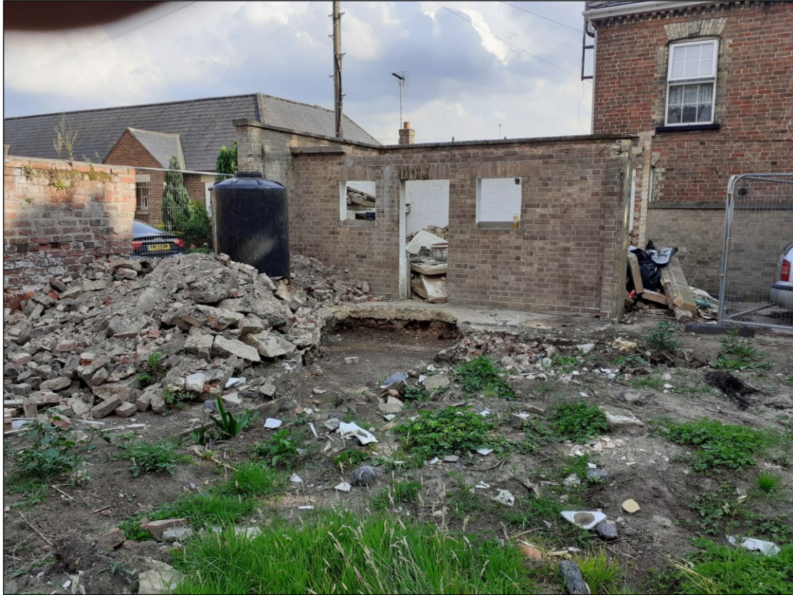
Plate 3: Area of Trench prior to excavation, looking south-east
