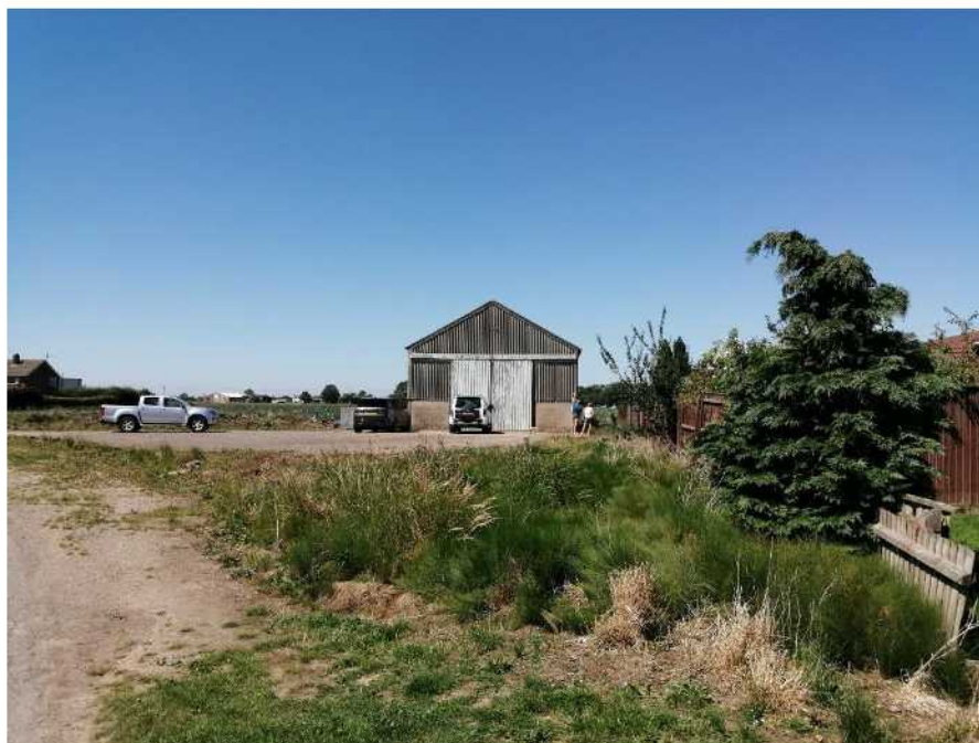
Front elevation of storage building
