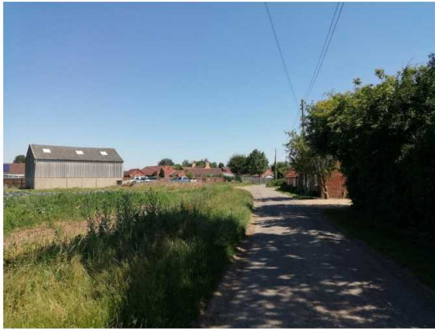
Side elevation of building viewed from site frontage
