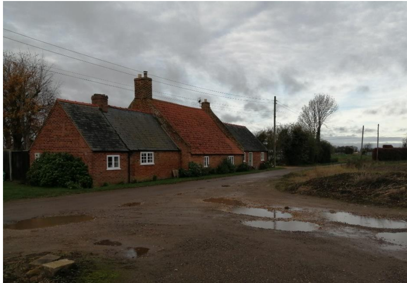
Photo of The Old Cottage as at November 2020
