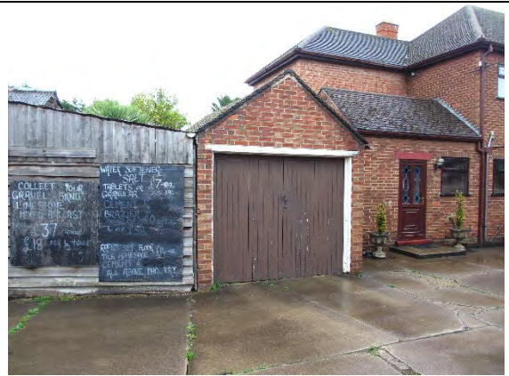
Photo 2: Rear of the dwelling with garage
