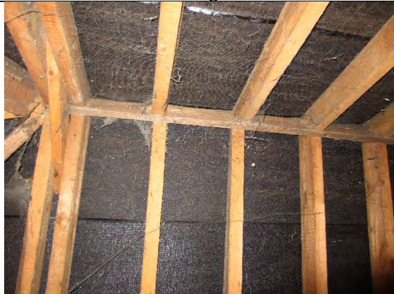
Photo 9: Cobwebs along ridge beam and rafters
