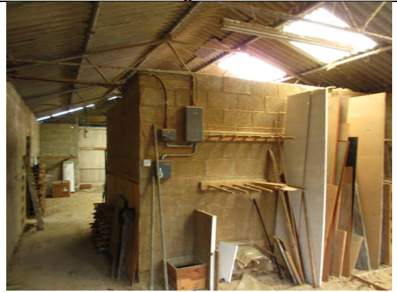
Photo 10: Typical exposed roof void in store/ workshop
