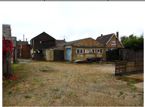
Photo 6: View West of Stores/ workshops near sales room
