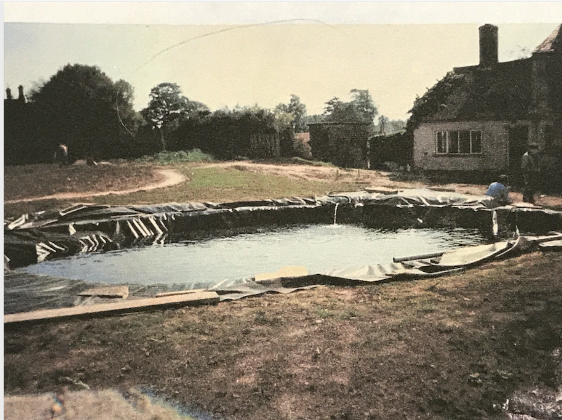
Pool being constructed during the 1970's
