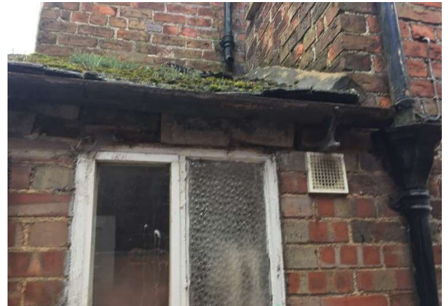
12. Window in right hand bedroom - to be repaired, remove rotten timber and replace in matching softwood.
