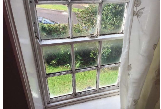
12. Window in right hand bedroom - to be repaired, remove rotten timber and replace in matching softwood.
