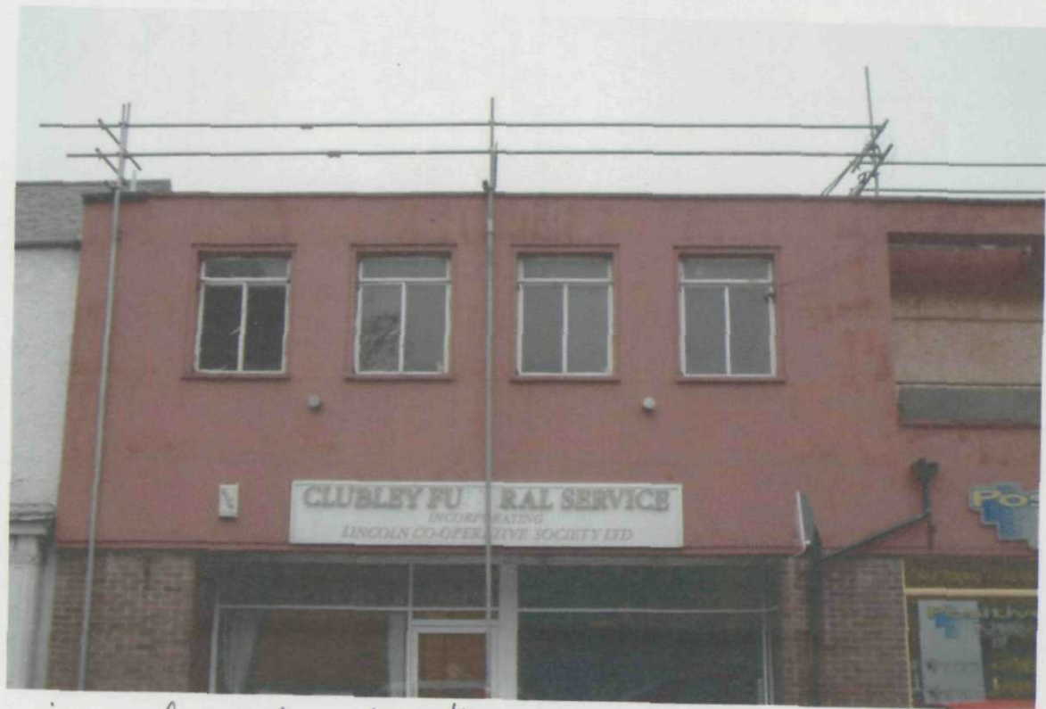
view of east elevation
