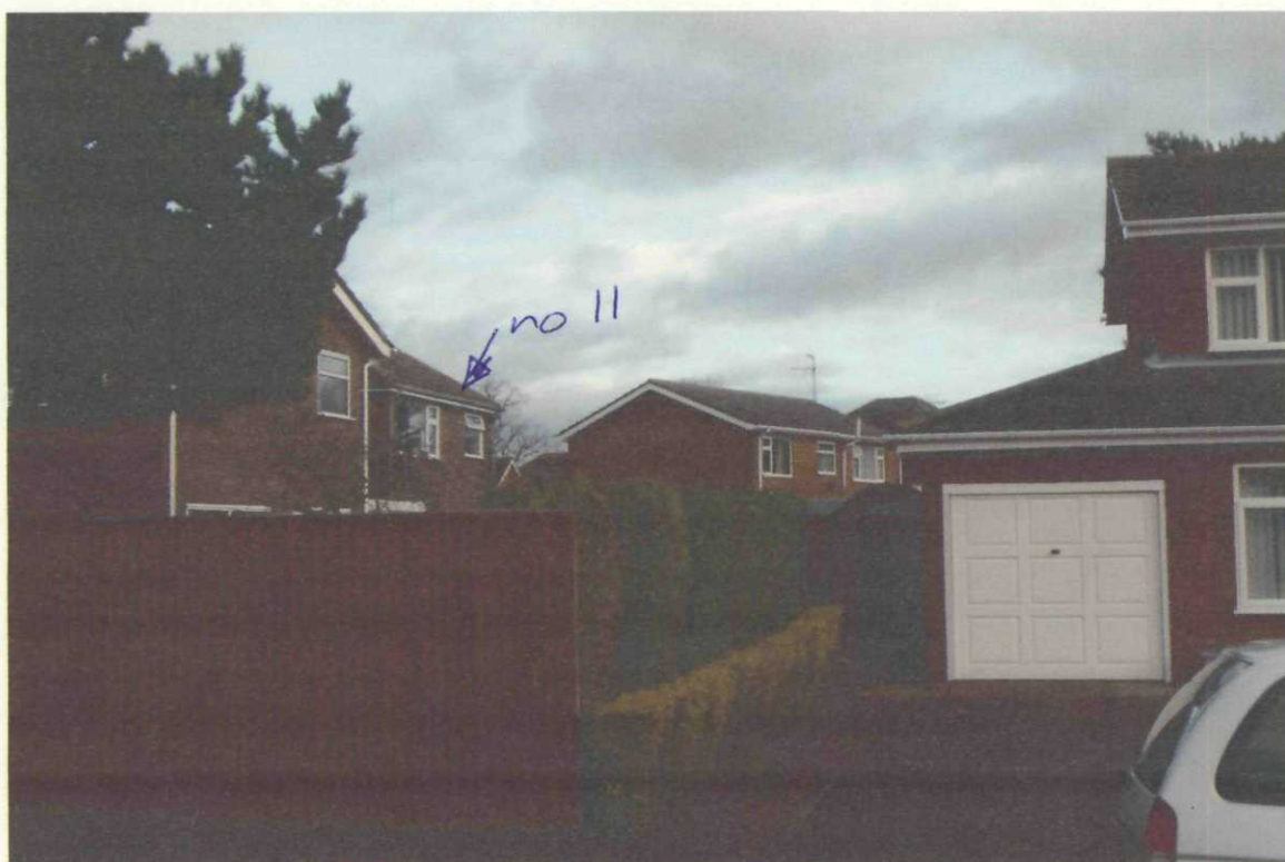
view from road looking east
