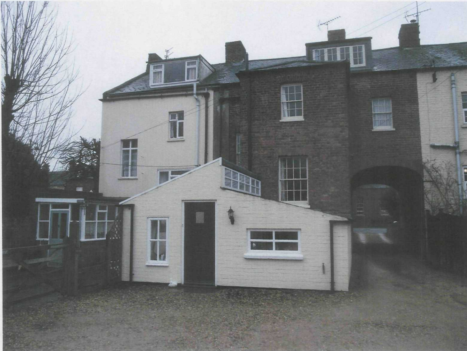
Rear view of neighbouring terrace 28 Market Street PE12 9DF
