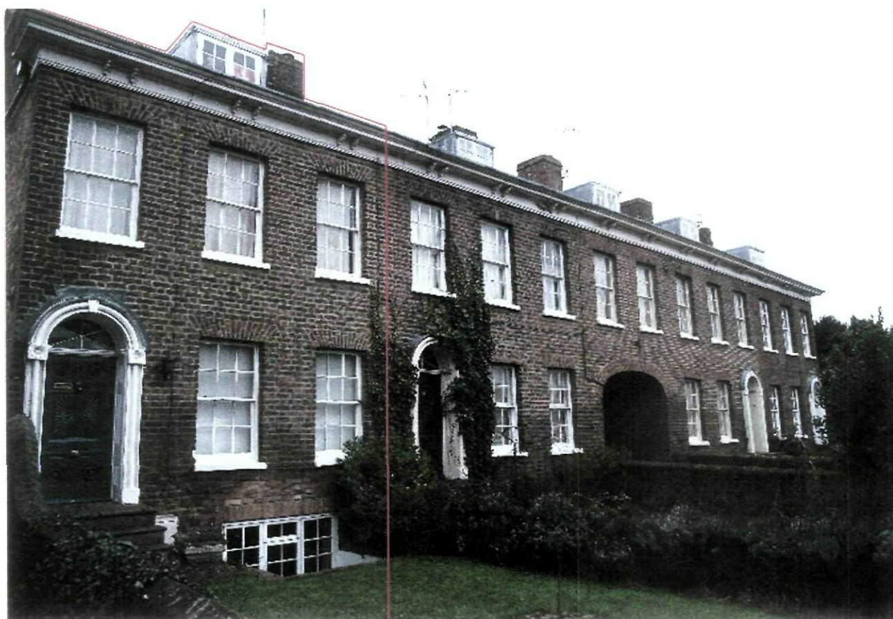
Front Elevation of 28 Market Street PE12 9DF
