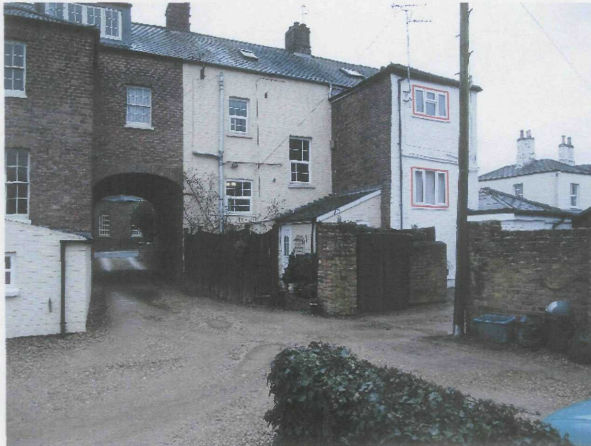
Rear Elevation of 28 Market Street PE12 9DF. 2 x U-pvc windows marked with red border which can be seen from rear of terrace
